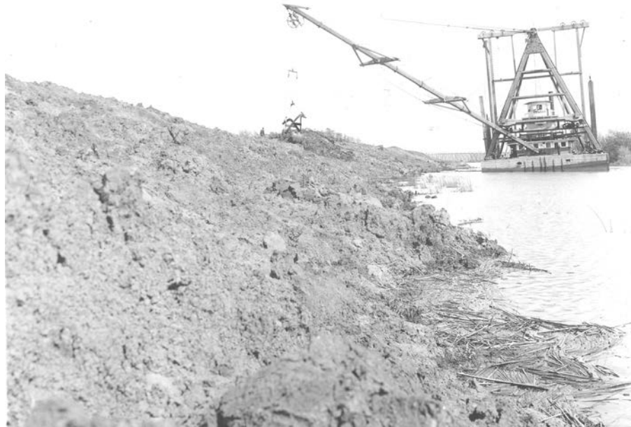
Figure 3-1: Dredge Vulcan Constructing Yolo Bypass Levee South of West Sacramento
