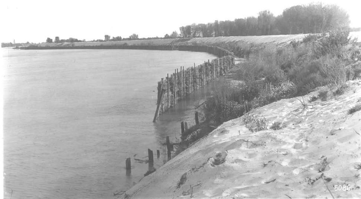
Figure 3-5: Levee Constructed Near Davis Road, West Sacramento
