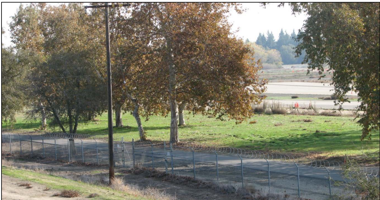
Figure 3.15-8. Looking Southeast Toward the CHP Academy.
