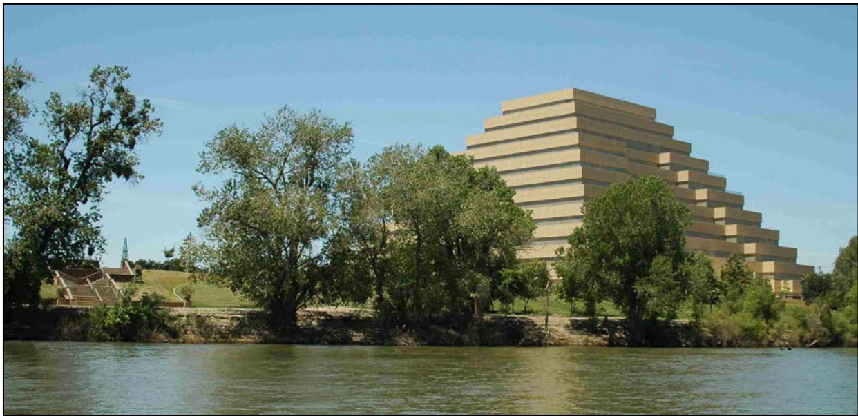
Figure 3.15-1. Looking Northwest Across the Sacramento River.
