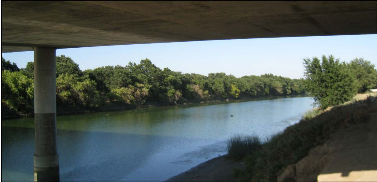
Figure 3.15-22. Looking East across the Barge Canal from the Port South Levee.
