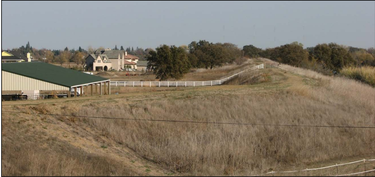
Figure 3.15-12. Looking West across the South Cross Levee.
