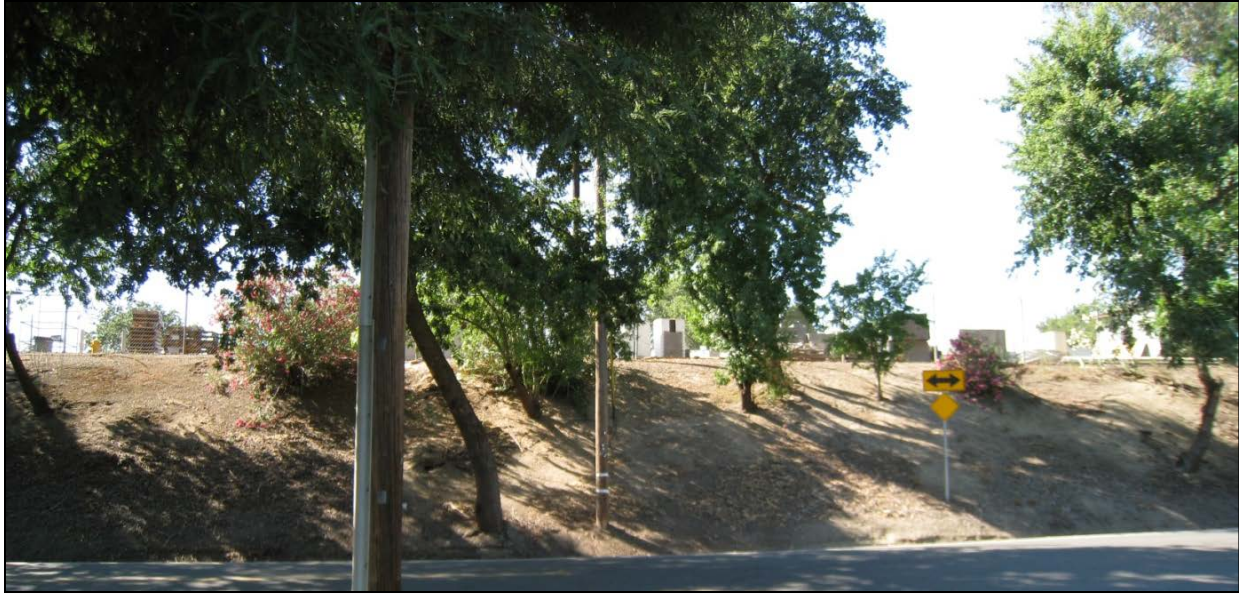
Figure 3.15-5. Looking North at the Sacramento River North Levee.
