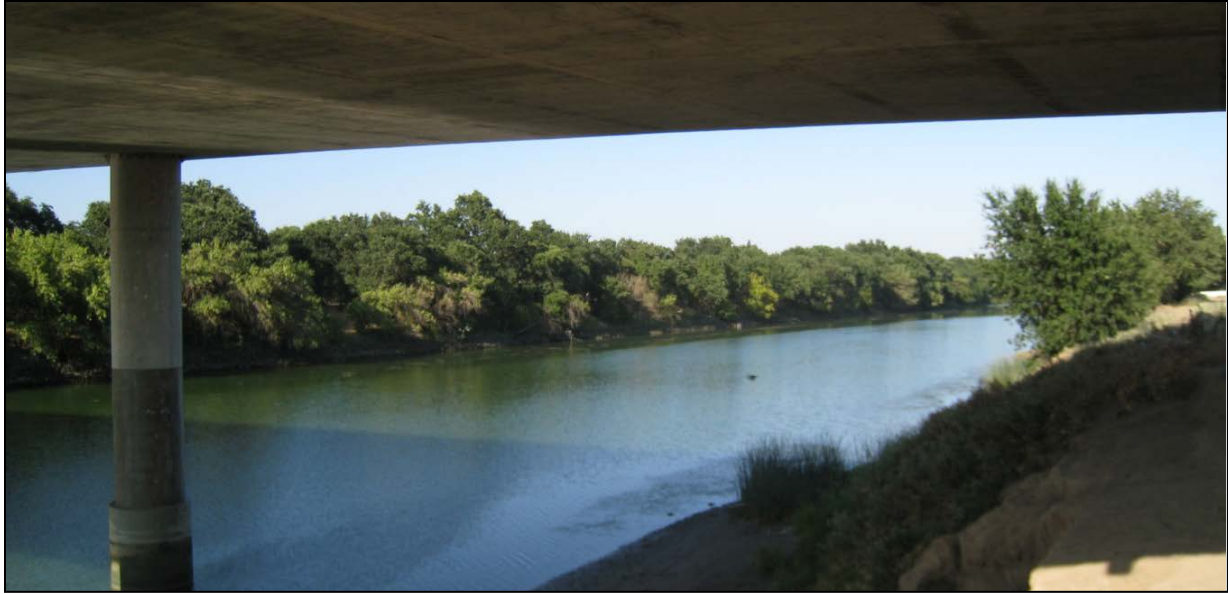
Figure 3.15-6. Looking East across the Barge Canal from the Port South Levee.
