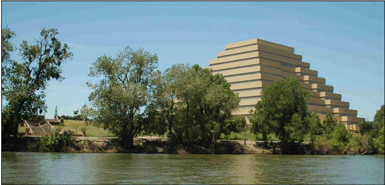
Figure 3.15-1. Looking Northwest Across the Sacramento River.
