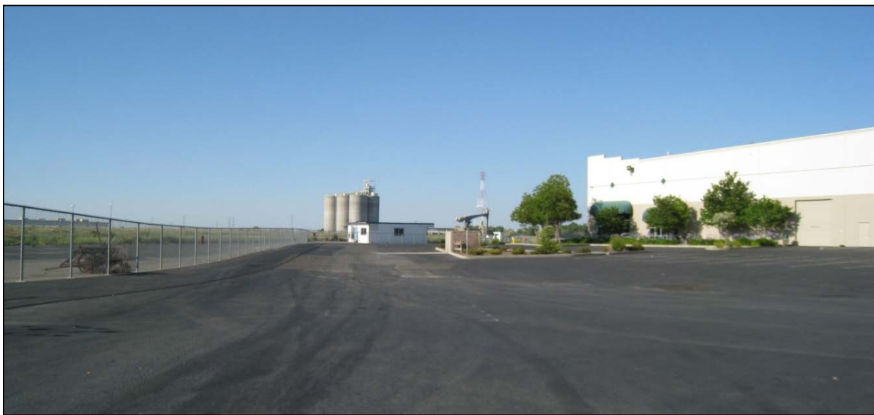
Figure 3.15-21. Looking Northeast at the Commercial Developments Adjacent to the Port South Reach.
