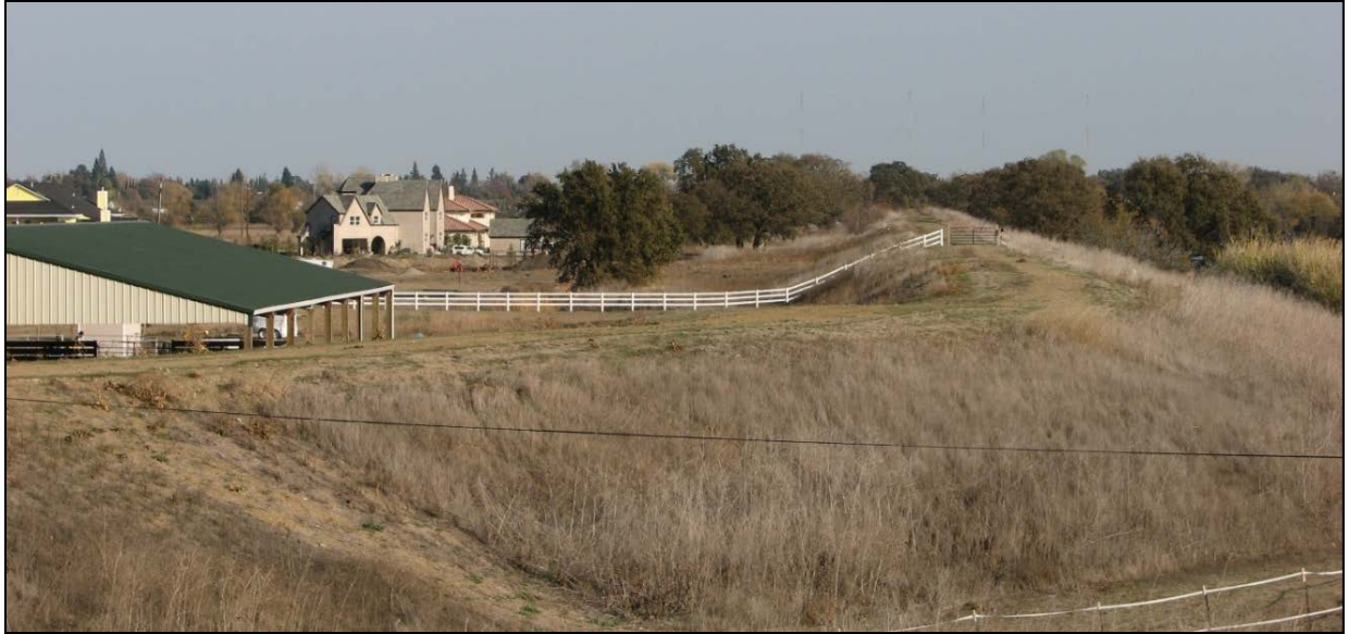
Figure 3.15-14. Looking West across the South Cross Levee.
