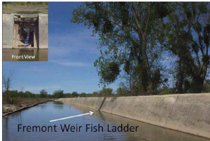
Figure 1-9 Fremont Weir Fish Ladder
