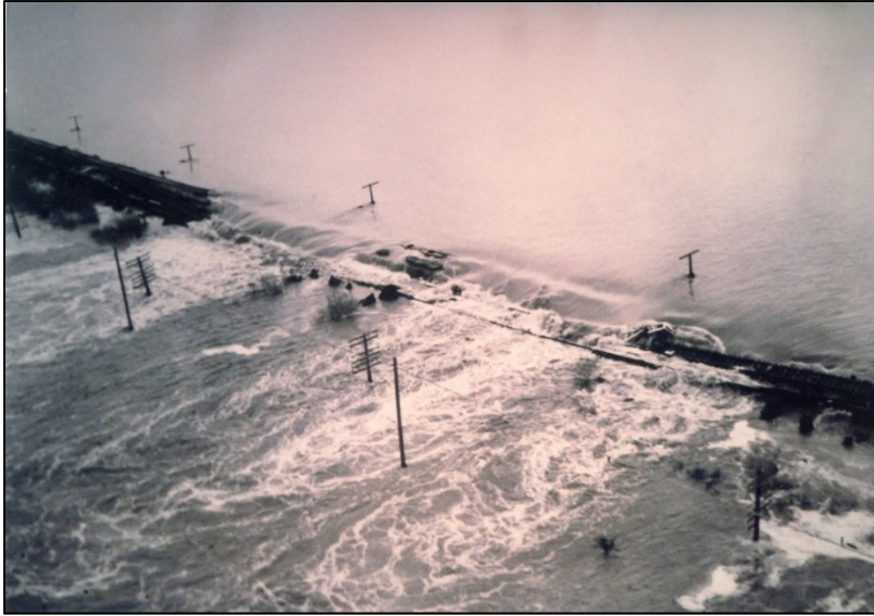
Figure 1-5 Levee Breach at Linda on Yuba River 1986
