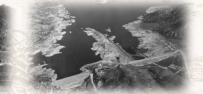
The completed Isabella Main Dam (left) and Auxiliary Dam (right), c. 1960.
