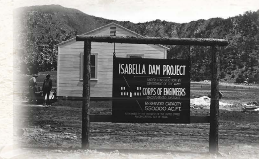
Isabella Dam project site, April 20, 1948.
