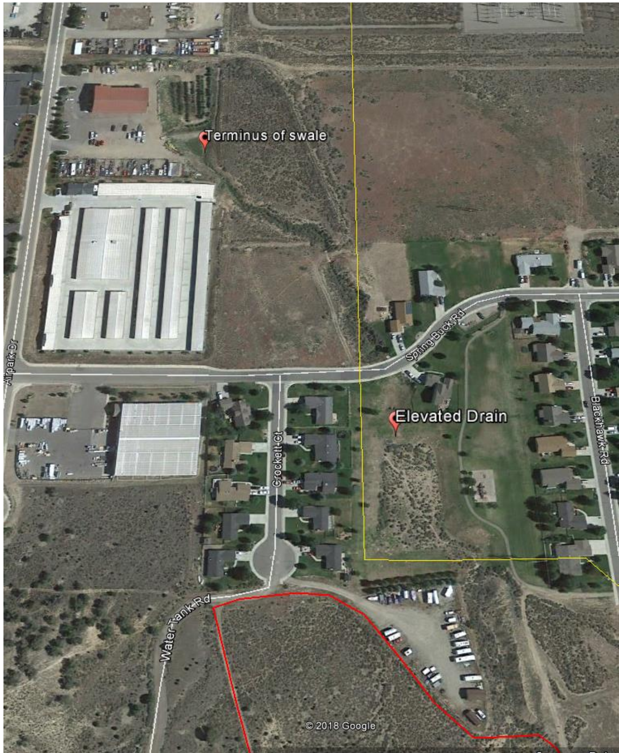
The elevated drain outlets to an upland swale north of Spring Buck Road, which terminates approximately 700 feet to the north as the slope flattens transitioning from foothills to floodplain.
