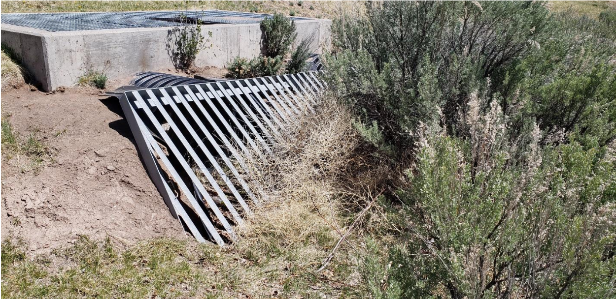
Elevated drain in detention basin
