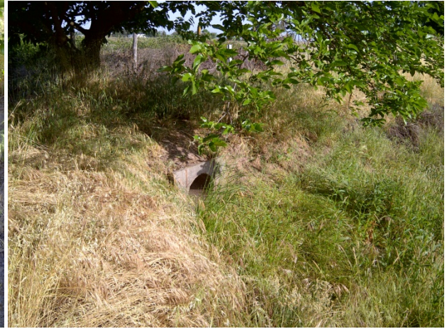
Photo 2 – The outfall of the culvert into the pond.
