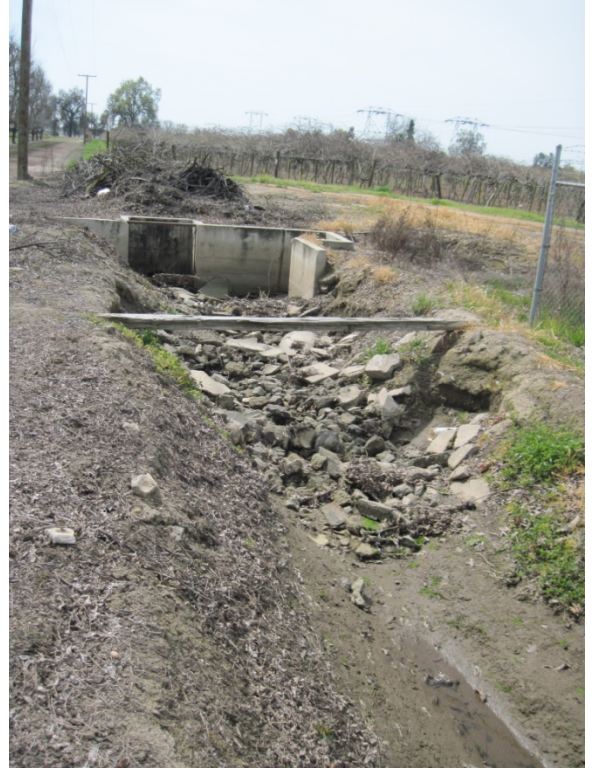
Downstream view of channel dcCH17
