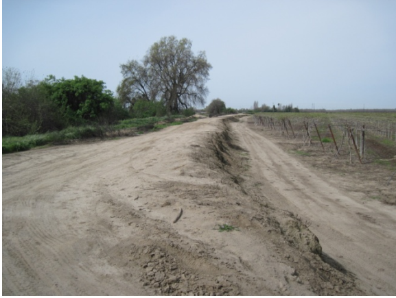
Levee outside the St. John's River
