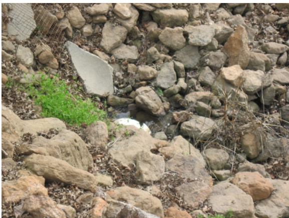
Small inlet pipe in pb30
