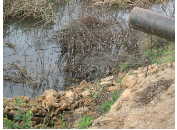
Close-up of outlet pipe
