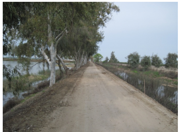
The levee between pb30 and dCH19
