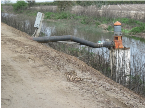
Pump taking water out of dCH19 for pb30
