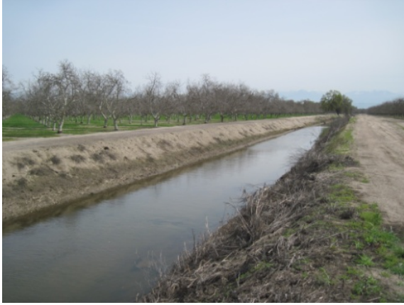
Upstream view of channel dcCH12 (Mill Creek)
