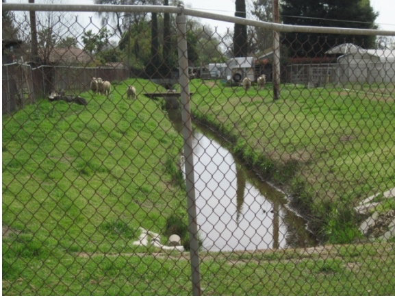
Upstream view of channel dcCH10
