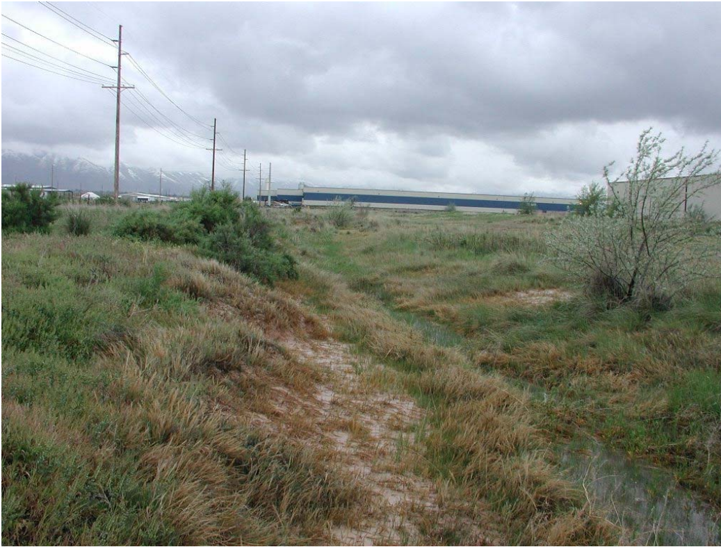
Photo 5: Picture of drainage swale looking south – up gradient
