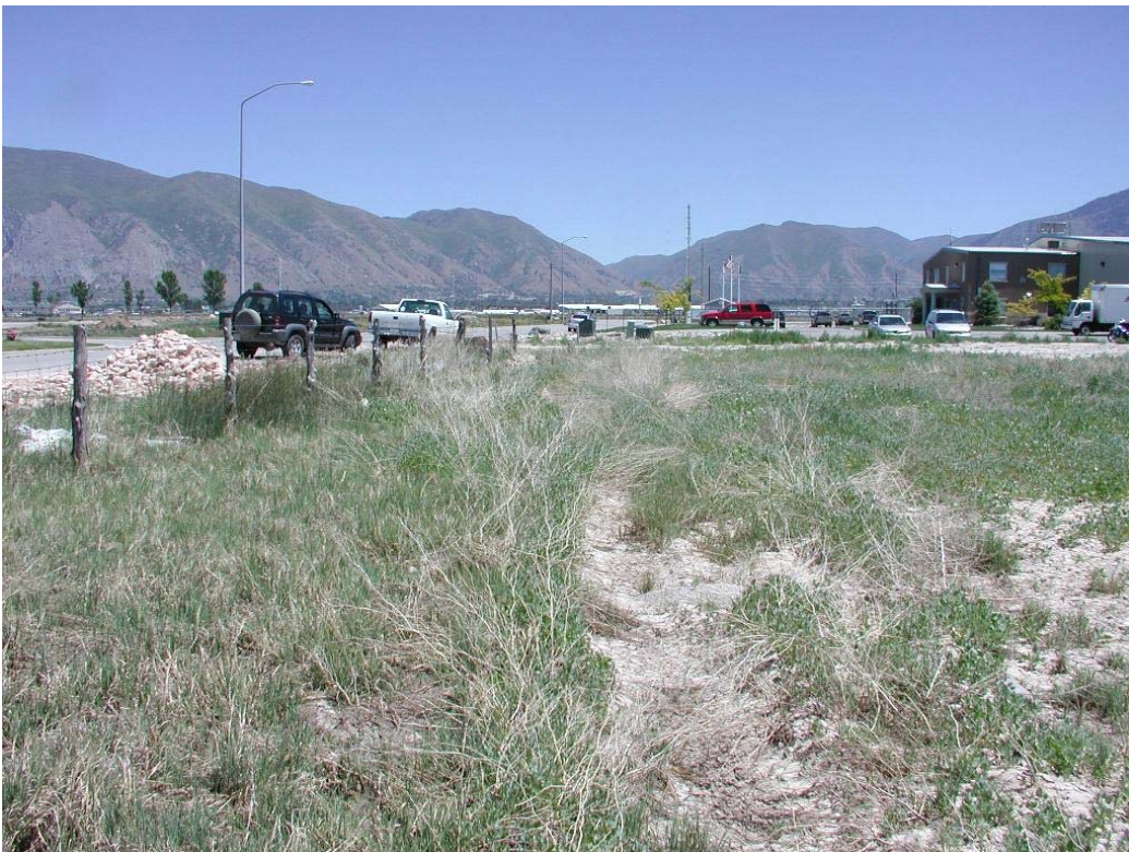
W10 (isolate) – Looking east along 3000 North Street. The eastern wetland boundary is located near the darker stand of juncus along the fence. The nearest connection to a RPW is the catch basin located approximately 50 feet in front of the white truck.
