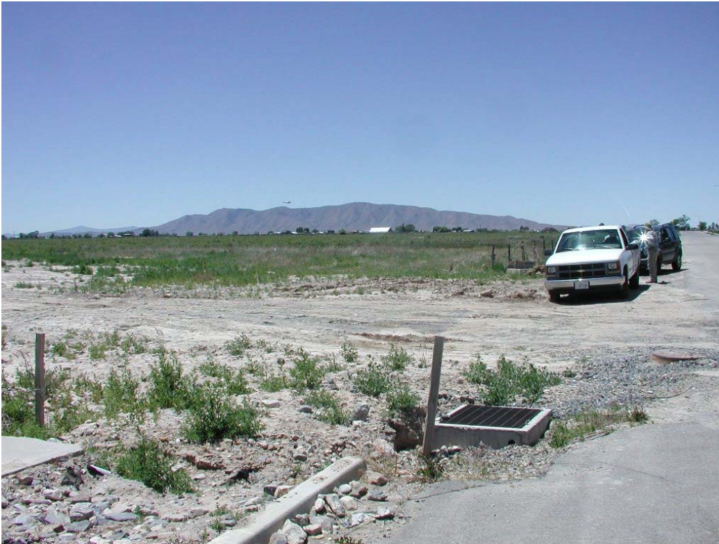
W10 (isolate) – Looking west along 3000 North Street. This catch basin is the only possible connection to a RPW. Runoff water would have to pond in W10 at least 2 feet in order to flow into the catch basin. The wetland boundary begins 6 fence posts west from the end post.
