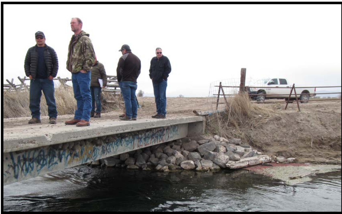
USACE staff looks at bridge riprap with tribal members
