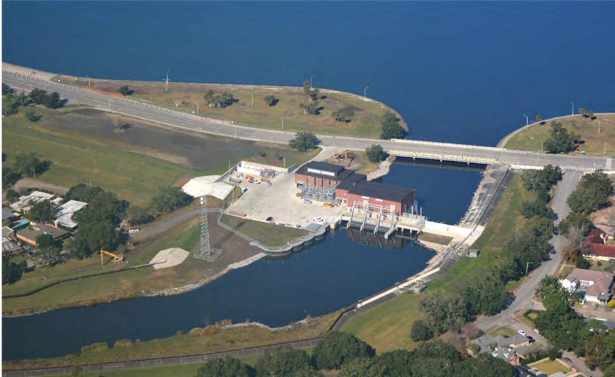
Figure 3.3. Station Intake Located on an Open Ponding Area, Orleans Ave. Pump Station Louisiana
