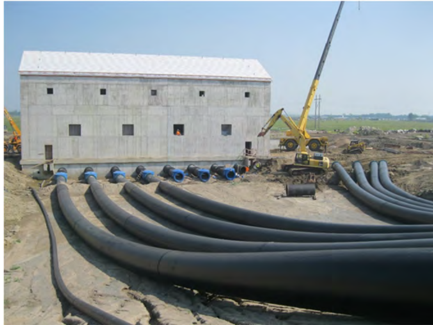
Figure 8.6. HDPE Discharge Pipe Installation, East Ditch Station North Dakota
