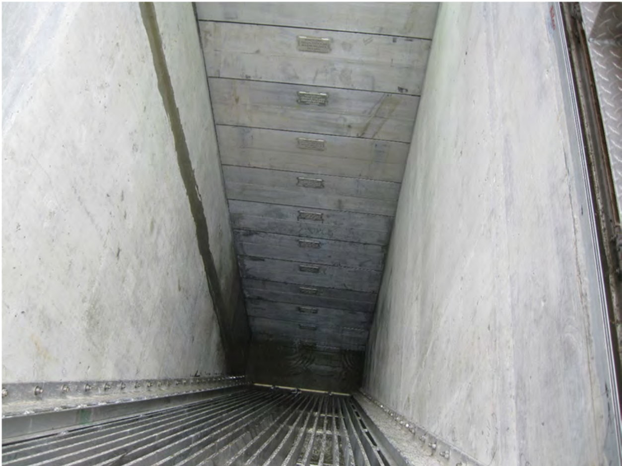
Figure 14.1. Stop Log Closure
