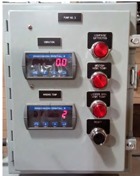
Figure 22.6. Separate Pump Protection
