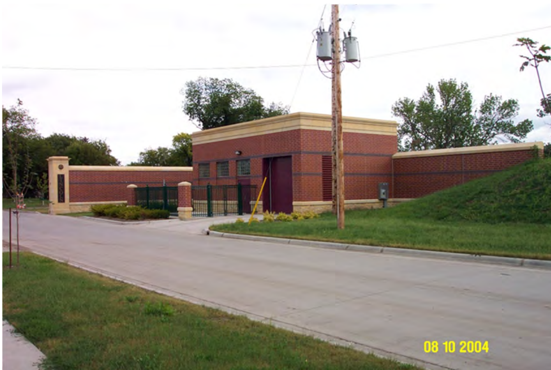
Figure 3.1. Flood Risk Management Drainage Station built into a floodwall
