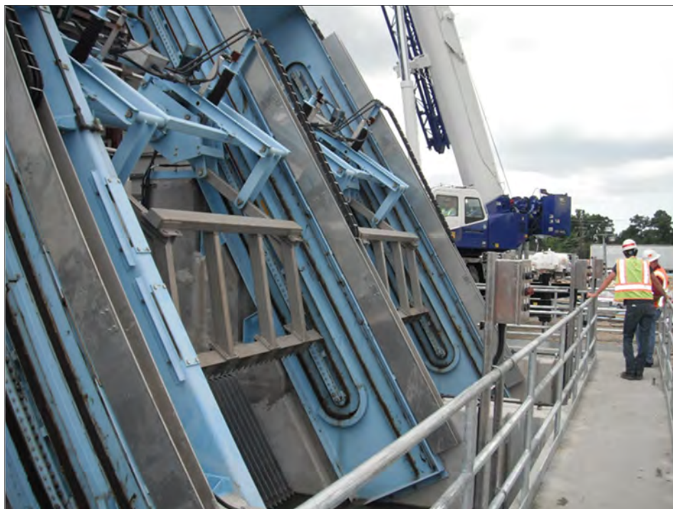
Figure 13.5. Mechanical Climber Screen Arrangement
