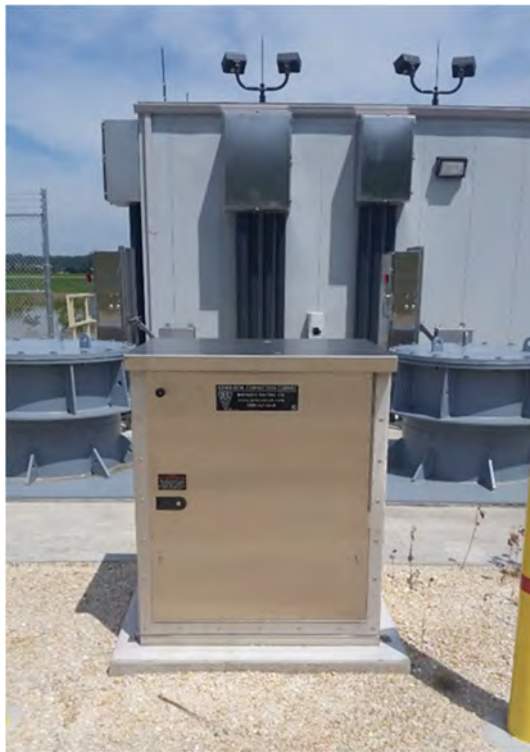
Figure 29.2. Generator Connection Enclosure
