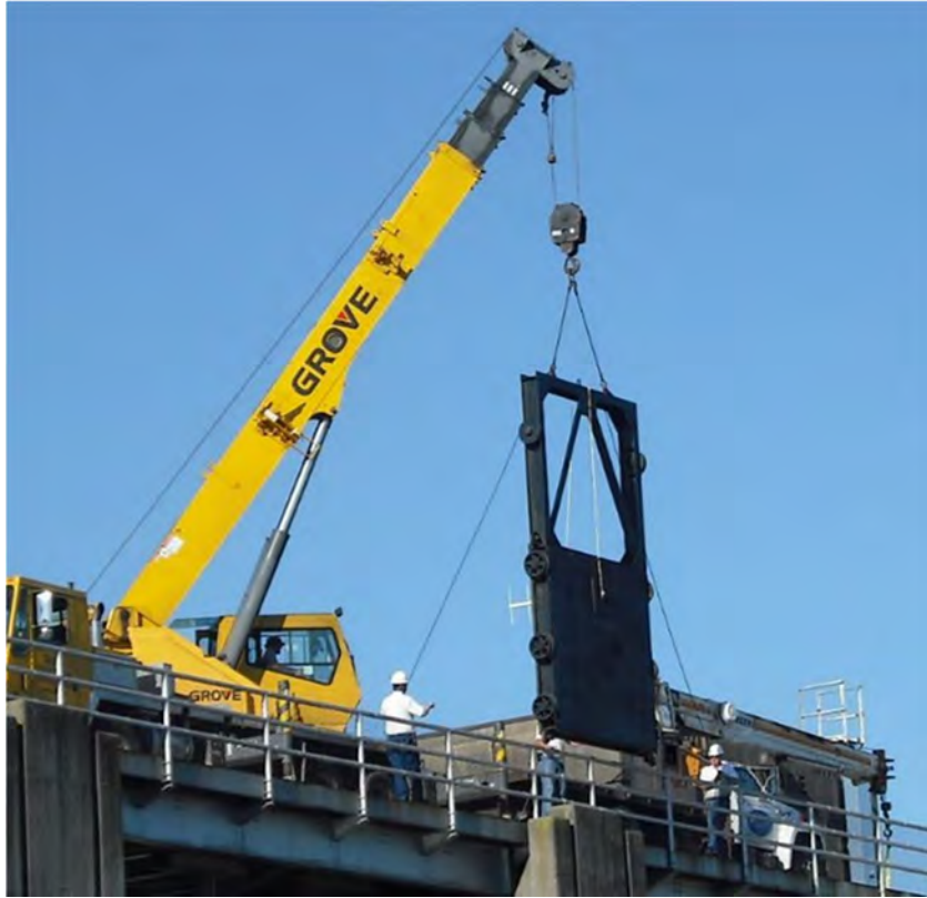
Figure 14.2. Bulkhead Placement
