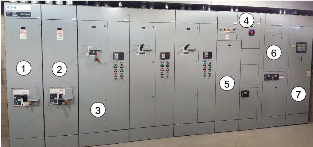
Figure 22.7. Pump Station MCC Integration
