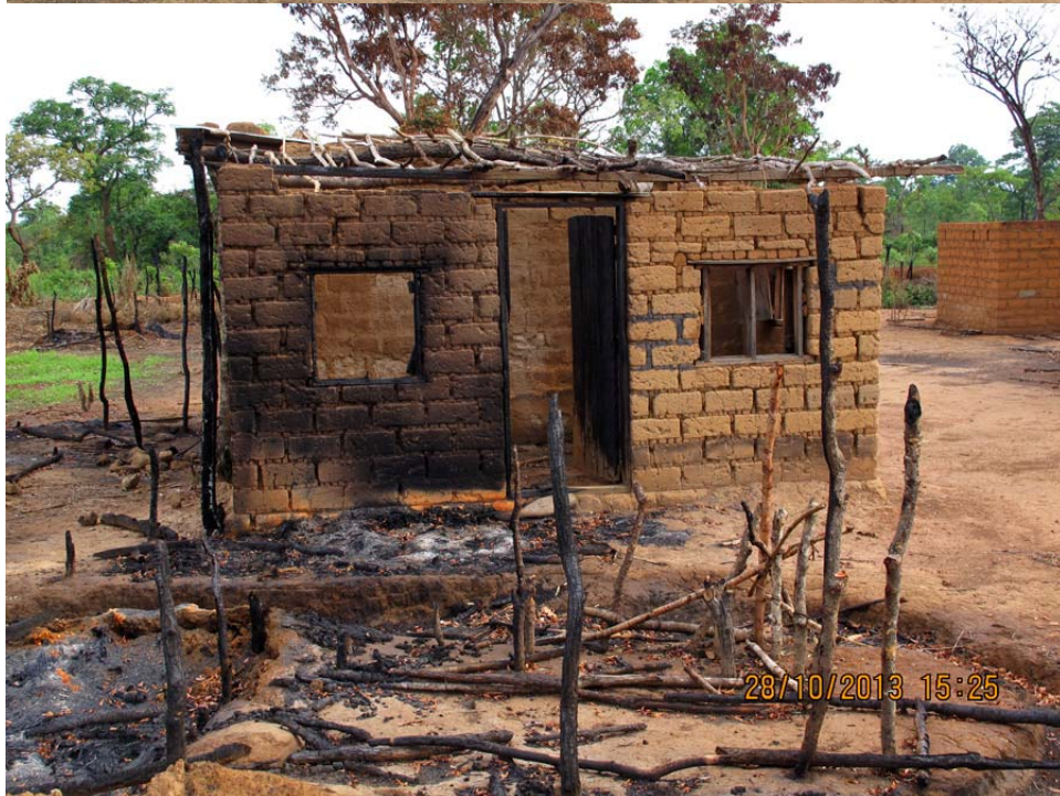
Burned structures in Kabola village.
