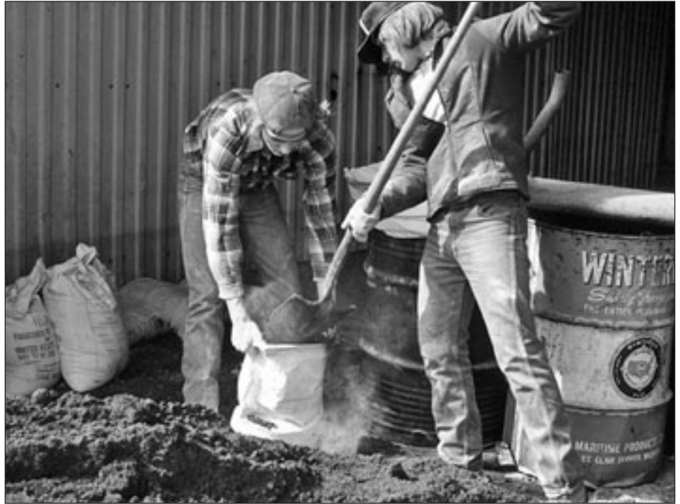
Filling sandbags for flood-fighting
