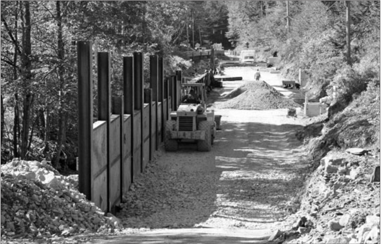
Construction of a streambank erosion control project along Basket Creek in Sullivan County, N.Y.
