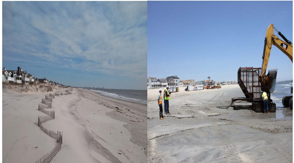
Preconstruction & during construction
