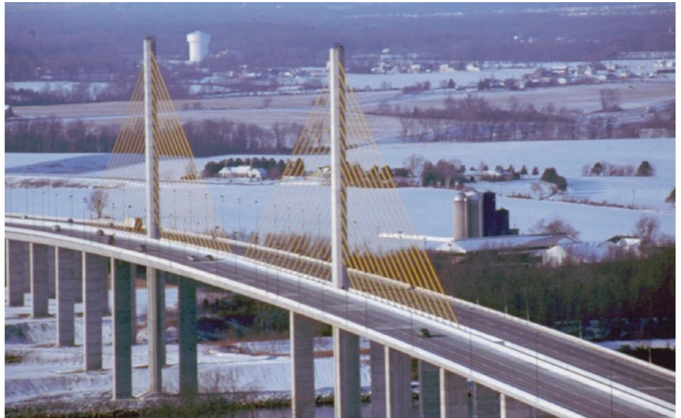
Senator Roth Bridge (SR-1) carrying roughly 34 million vehicles over the C&D Canal per year. Operated and Maintained by USACE Philadelphia District.
