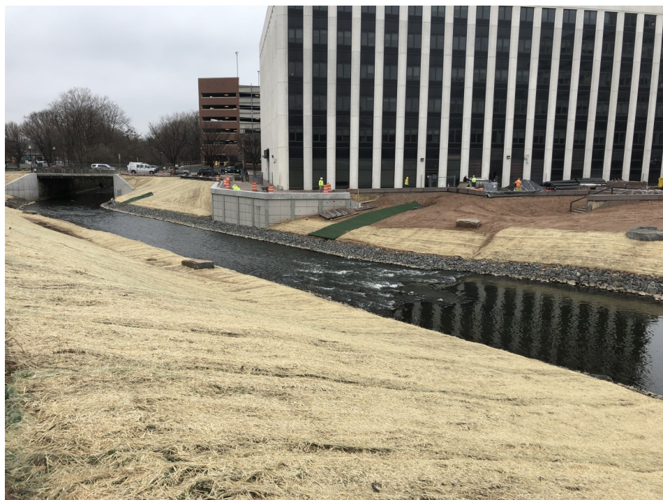
Upstream view of restored stream channel prior to planting of native vegetation scheduled for spring 2020.
