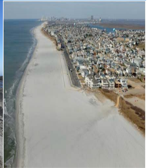
Right: Aerial Photo of the Completed Storm Damage Reduction Beach fill – Brigantine Island.
