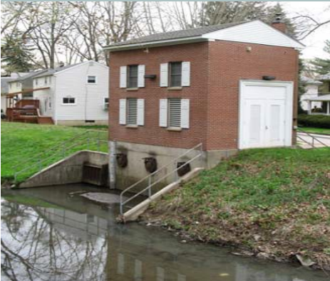
A pump house along Tookany Creek in Cheltenham drains water from the leeward side of the levee into the main channel. However, during period of high flow, the water has no where to drain.
