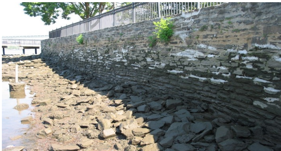
View of seawall with recent local repairs
