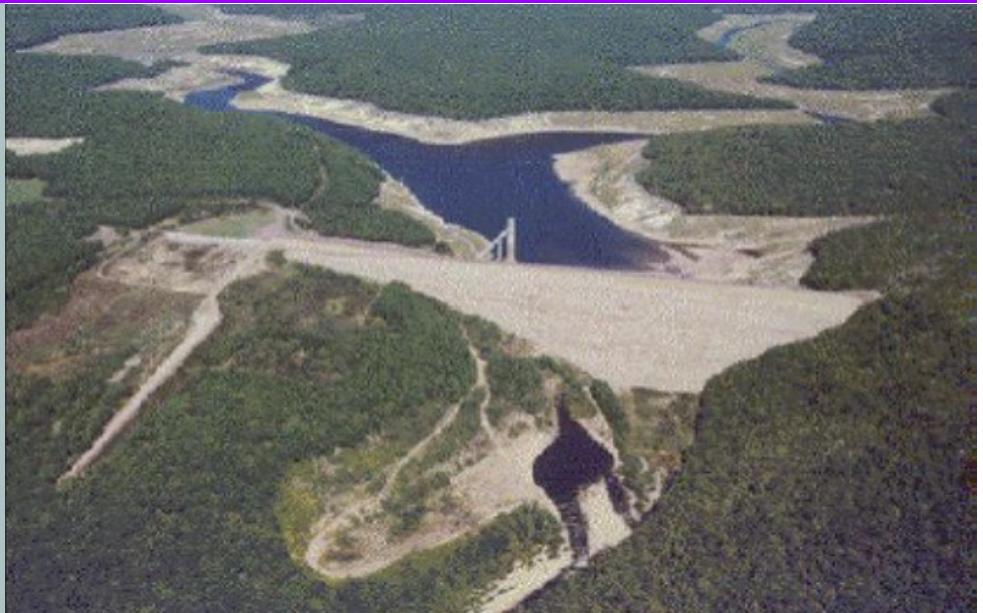
Francis E. Walter Dam and Reservoir
