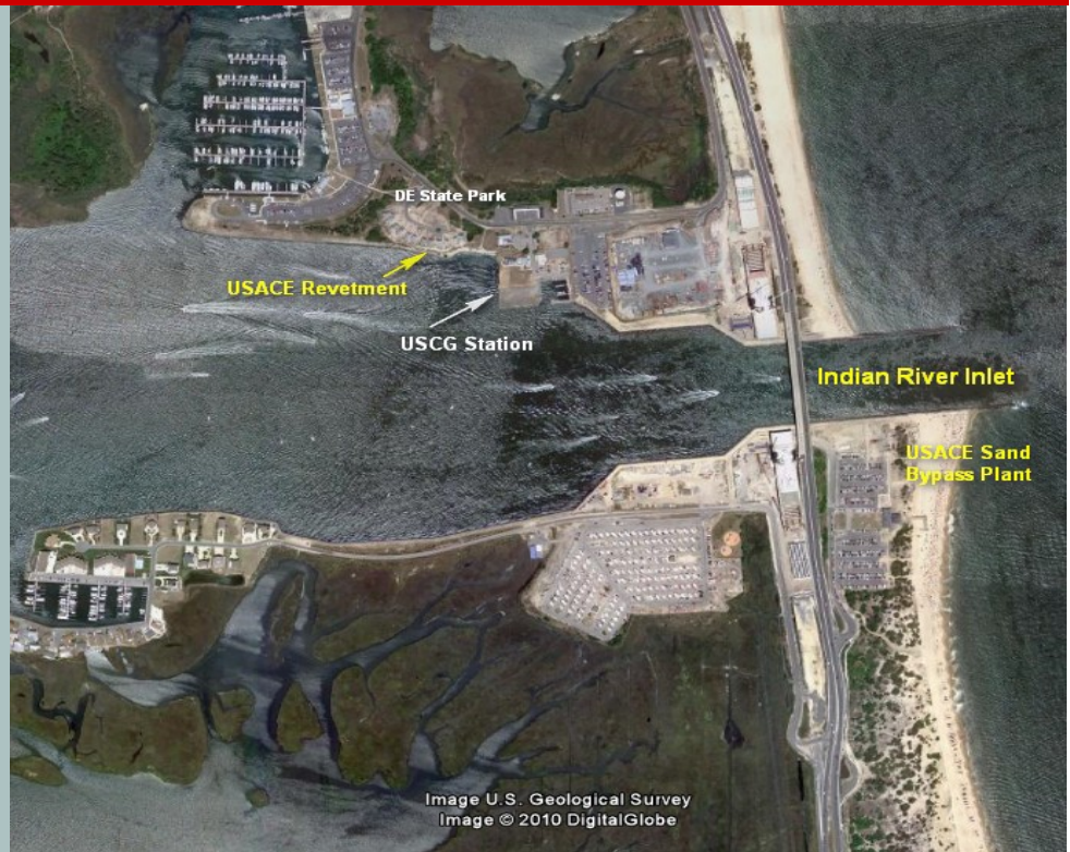
Aerial view of project area showing Indian River Inlet.
