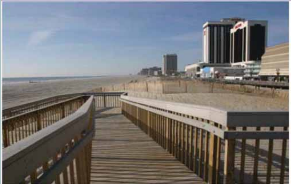
Absecon Island - Completed Handicap Dune Crossing.
