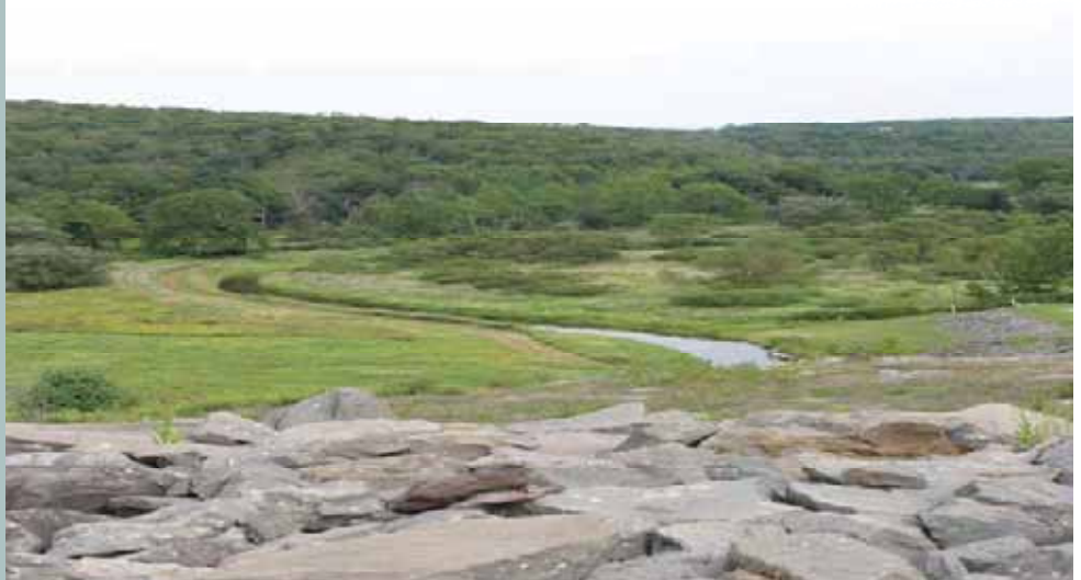
Dyberry Creek at base of General Jadwin Dam.
