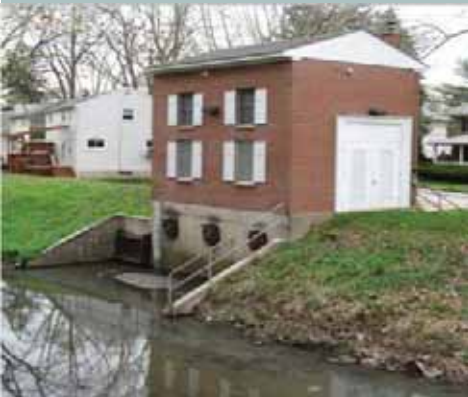
A pump house along Tookany Creek in Cheltenham drains water from the leeward side of the levee into the main channel. However, during period of high flow, the water has no where to drain.
