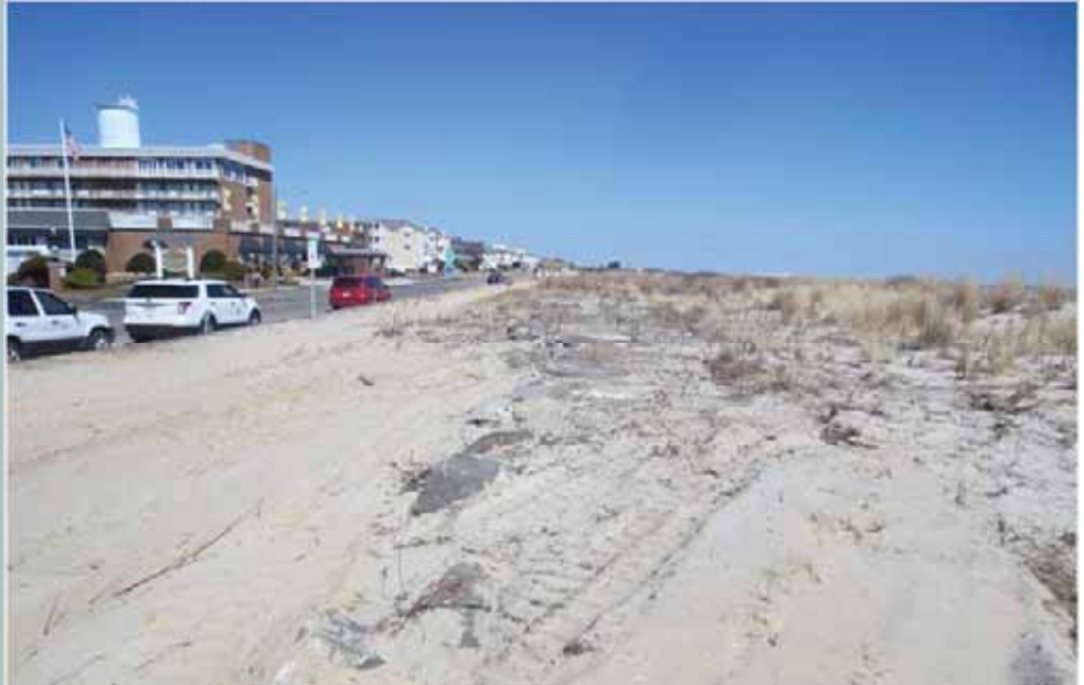
Existing seawall that is located between Beach Avenue and the beach on the south side of the City of Cape May.
