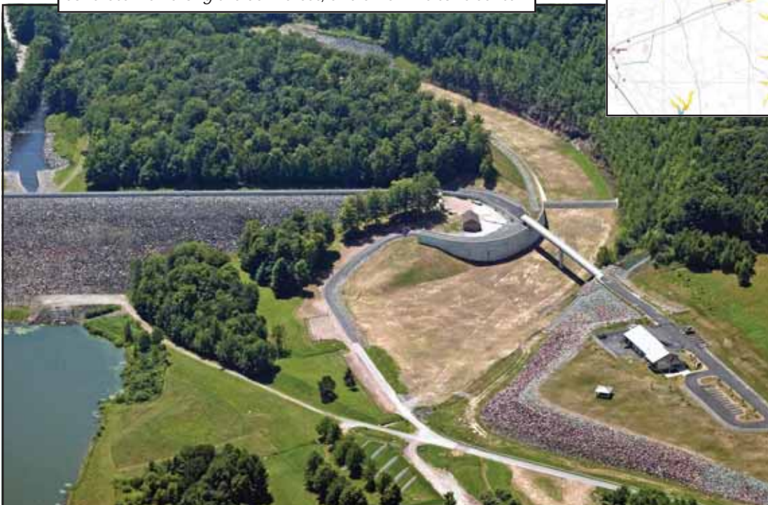
Prompton Lake, Lackawaxen River Basin, PA: Recent major modifications included an enlarged spillway, a protective concrete wall along the dam crest, and a new visitor's center.
