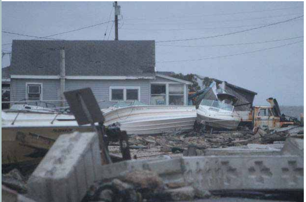
Damages from Hurricane Sandy along the Delaware Bay at Gandys Beach in Downe Township.
