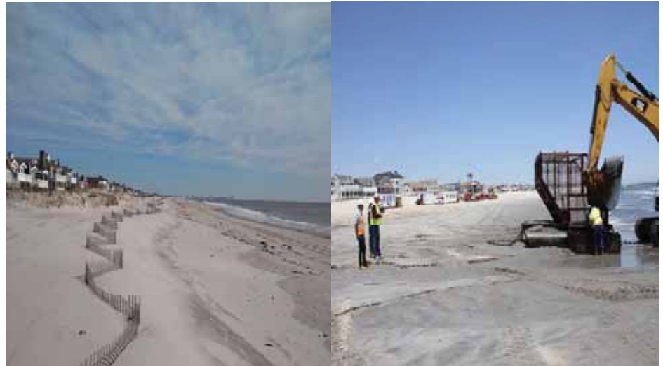
Preconstruction & during construction
