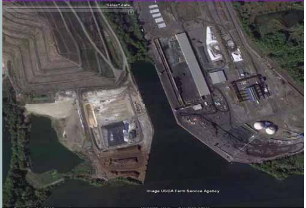
Port of Bucks County—Fairless Turning Basin
