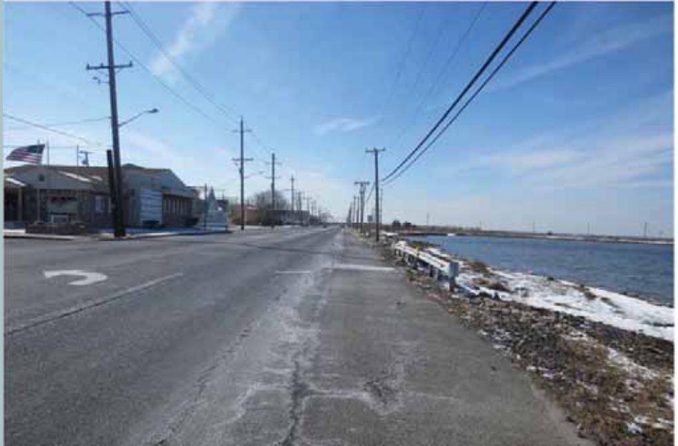
West End Avenue on the north side of Chelsea Heights is frequently flooded by the bay behind Absecon Island.
