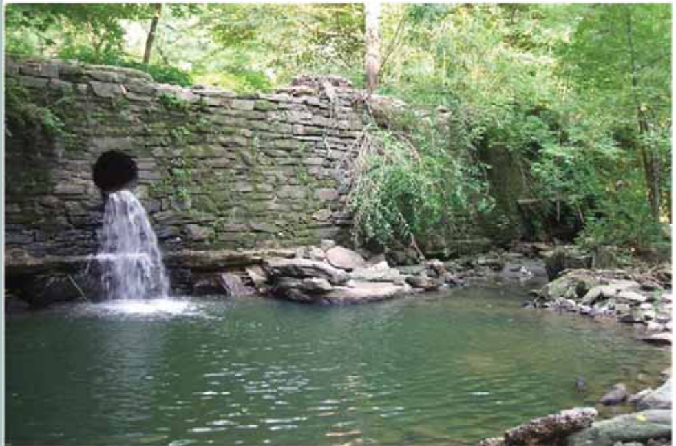
Upstream view of Cresheim Dam
