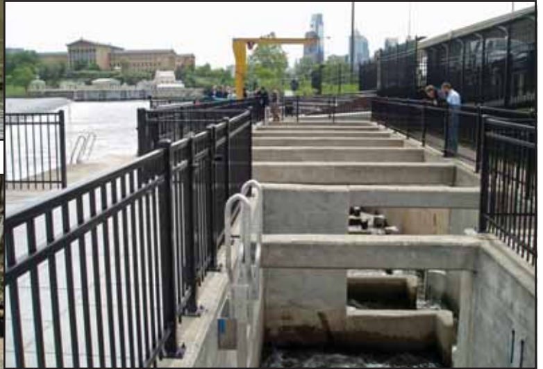
Fairmount Dam Fish Ladder, Philadelphia, PA: The District upgraded a 1970s-era structure to allow more shad and other migratory fish to swim upstream the Schuylkill River.
