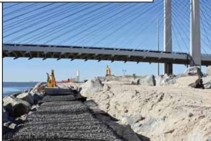
Indian River Inlet, DE: Post-Sandy work to reinforce the north jetty involved placing marine mattresses, filling voids and positioning capstones.
