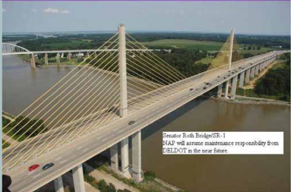
Senator Roth Bridge (SR-1). Philadelphia District will assume maintenance responsibility from DEL DOT in the near future.
