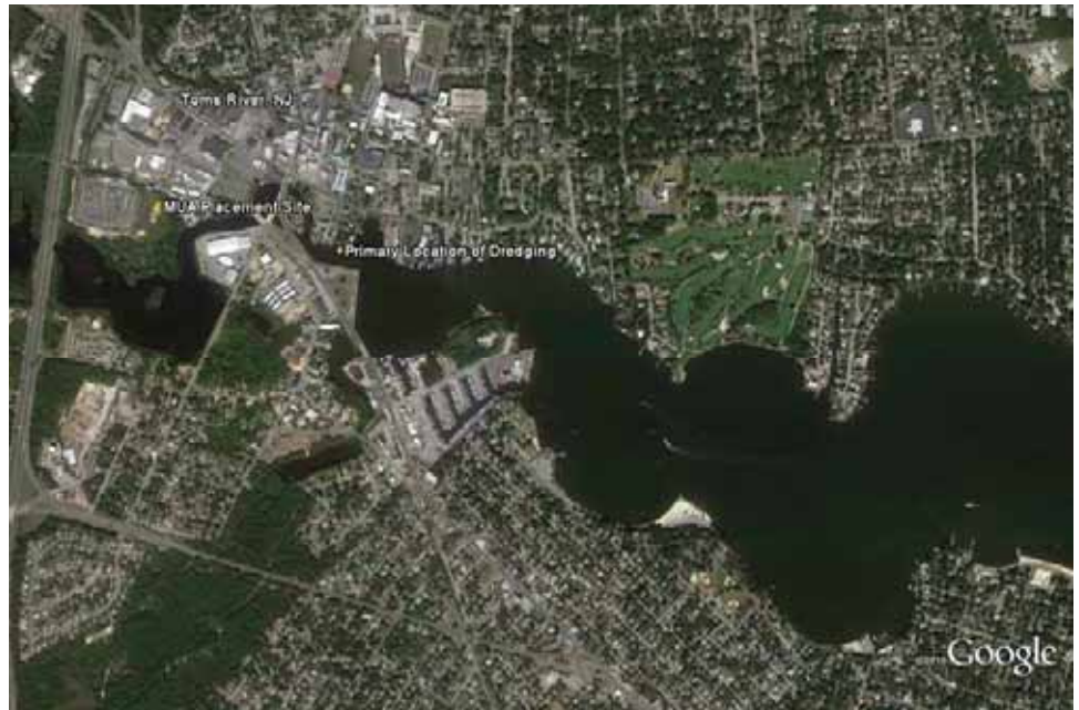
Aerial view of project area—Toms River, NJ
