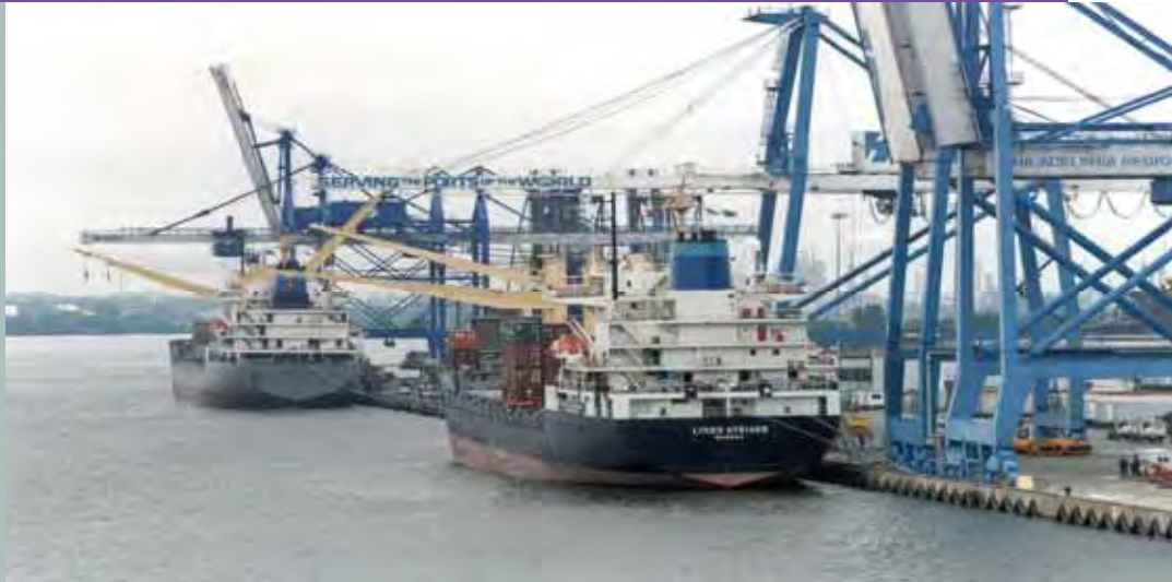
Container Vessels being unloaded at Port of Philadelphia
