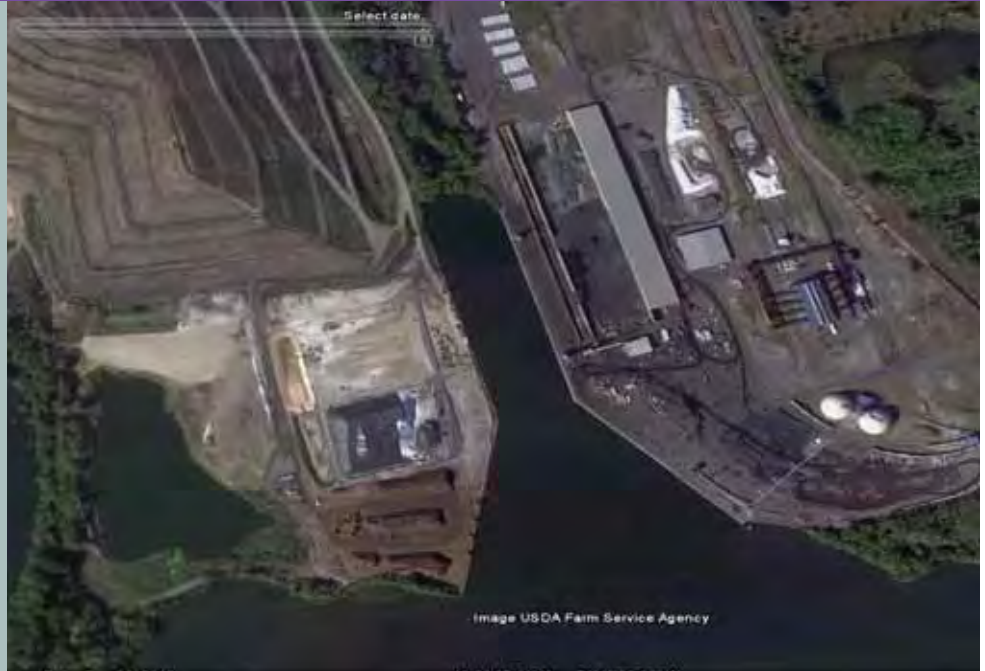
Port of Bucks County—Fairless Turning Basin
