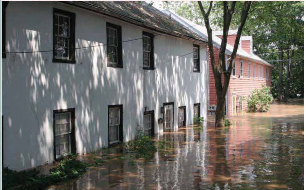
1st floor flooding of residential structures in New Hope, PA (June 2006).
