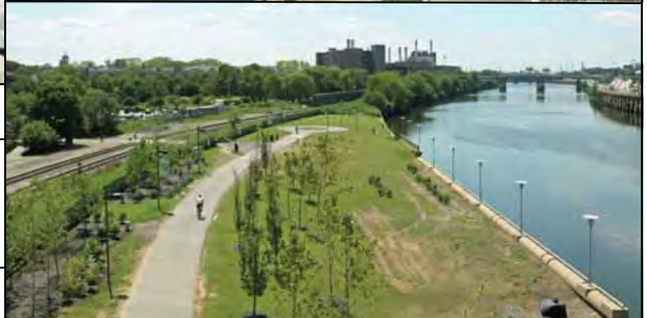
Schuylkill River Park, Philadelphia, PA: Construction of this multi-use linear park added highly visible and accessible green space in the heart of the city.
