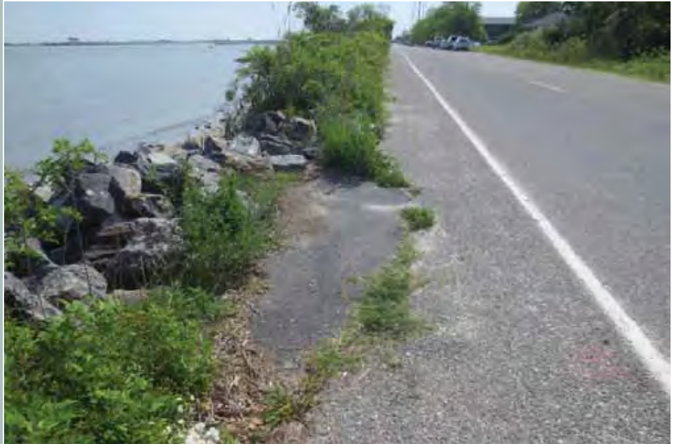
Delaware Avenue in the City of Cape May is threatened by erosive forces from Cape May Harbor.
