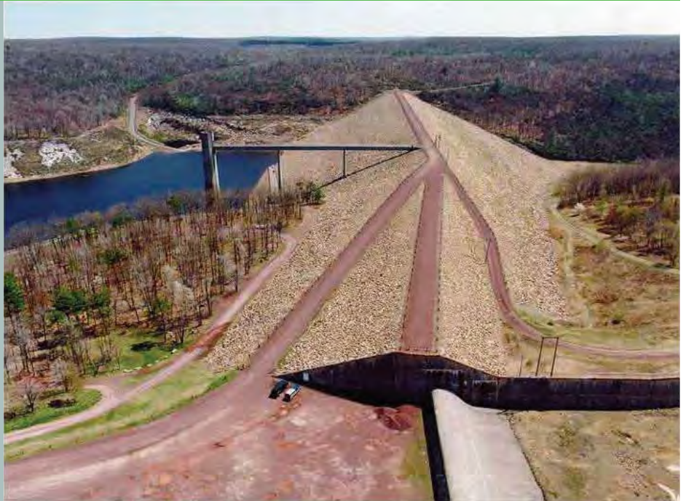
The existing project, initially constructed in 1961, provides for multipurpose development for water supply, recreation and flood control. The project is located on the Lehigh River, five miles above White Haven, Pa.
