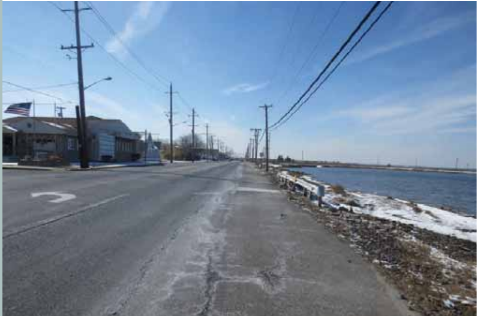
West End Avenue on the north side of Chelsea Heights is frequently flooded by the bay behind Absecon Island.
