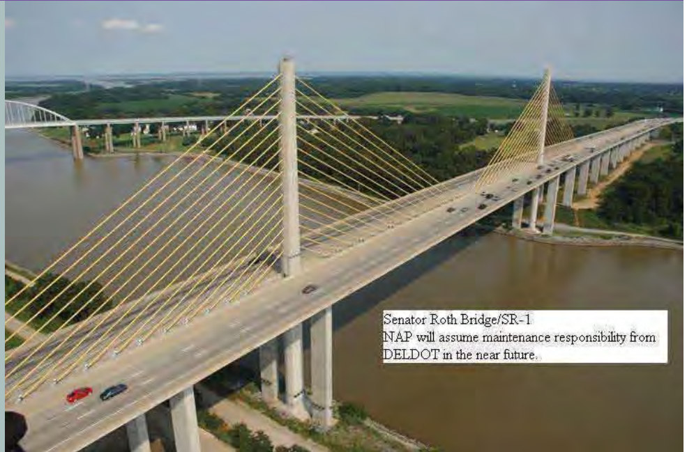
Senator Roth Bridge (SR-1). Philadelphia District will assume maintenance responsibility from DEL DOT in the near future.
