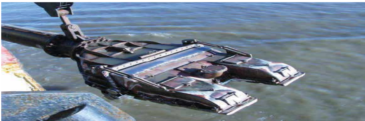
Dredging is accomplished by a drag arm on each side of the ship with a drag head at each end. As the ship navigates the channel with its dredging pumps engaged, the drag heads are lowered to the channel bottom. Like vacuum cleaners, they pull the dredged material into the ship's hoppers.
