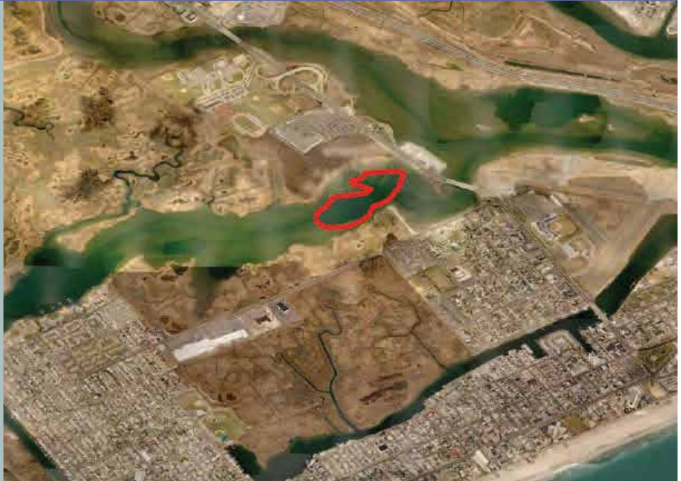
Aerial photograph depicting the project site for Dredged Hole 34 including the proposed dredged hole and dredged material locations.
