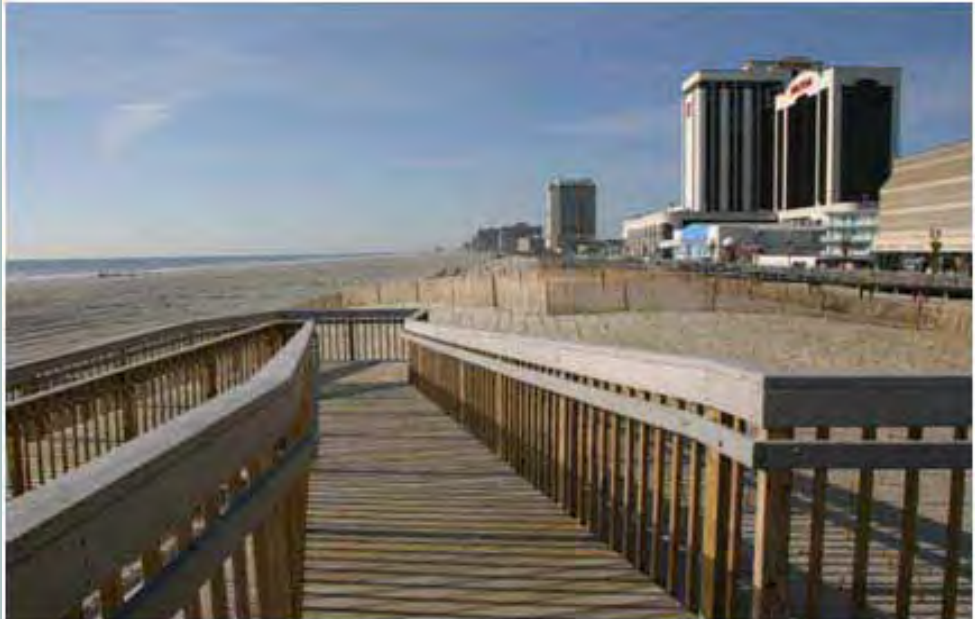
Absecon Island - Completed Handicap Dune Crossing.
