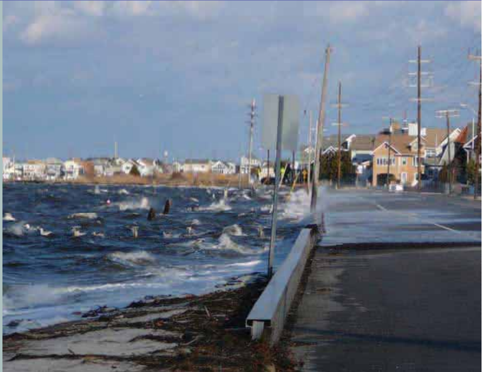
Bayside flood problems are a common issue in Barnegat Bay and tidal bays along New Jersey and Delaware. The solution is usually more complicated than ocean-front areas due to available land area.
