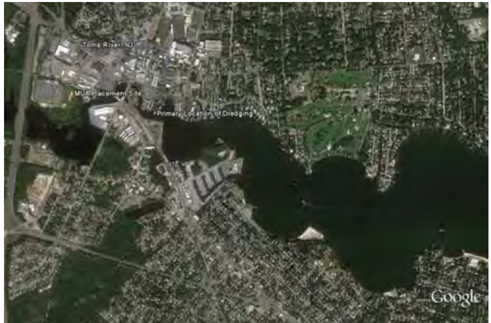
Aerial view of project area—Toms River, NJ
