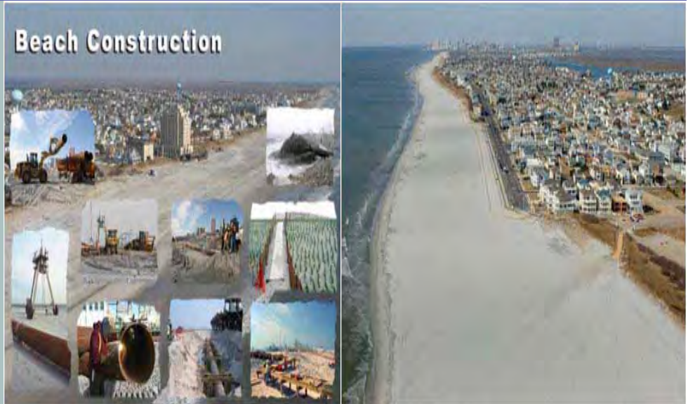
Left: Initial Storm Damage Reduction Beach Construction - Brigantine Island.
