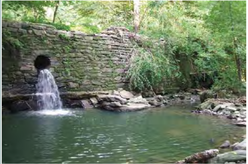
Upstream view of Cresheim Dam
