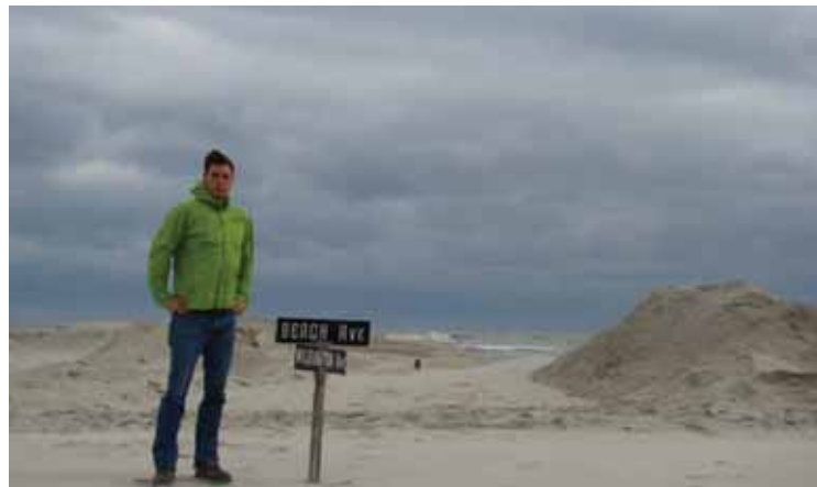
Approximately 6 feet of sand that was washed over the seawall and onto the street at the corner of Wilmington Avenue and Beach Avenue during Hurricane Sandy.
