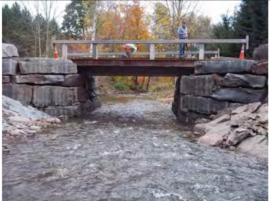
Inspection of small span bridge at Walton, NY
