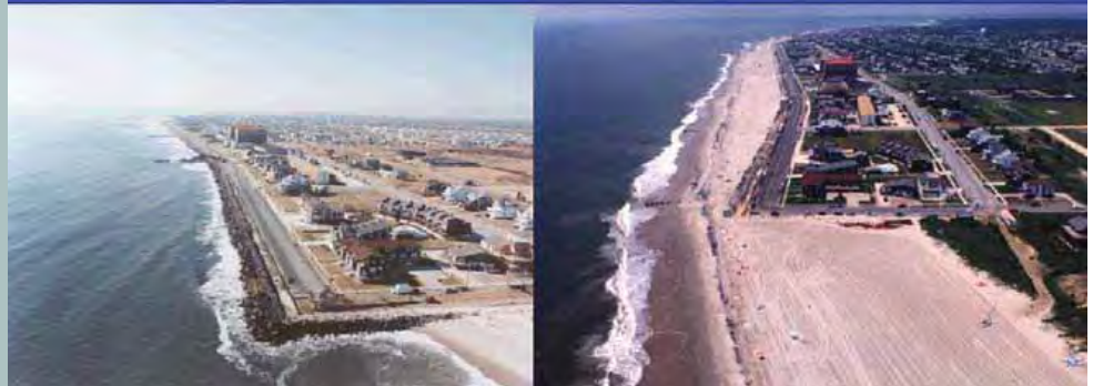
Completion of initial construction and continued periodic nourishment by the Corps maintains a beach in Cape May after it was lost to erosion over the years.
