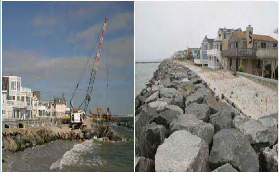
Left: Avalon Seawall During construction. Right: Avalon Seawall Completed Section
