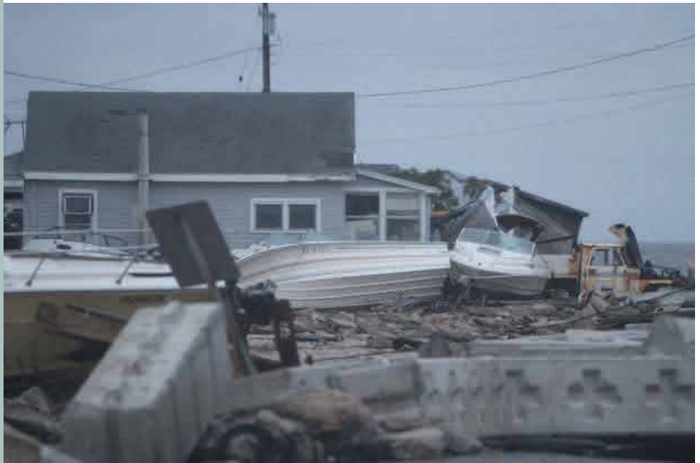
Damages from Hurricane Sandy along the Delaware Bay at Gandys Beach in Downe Township.
