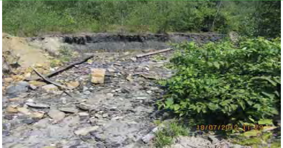
Former stream channel along the West Branch Schuylkill River. The stream now flows into underground mines .
