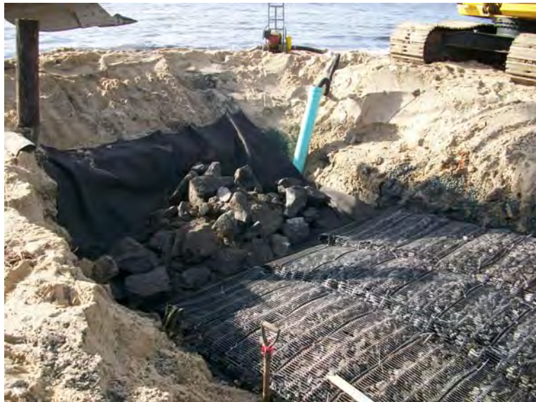
Marine mattresses under construction.
