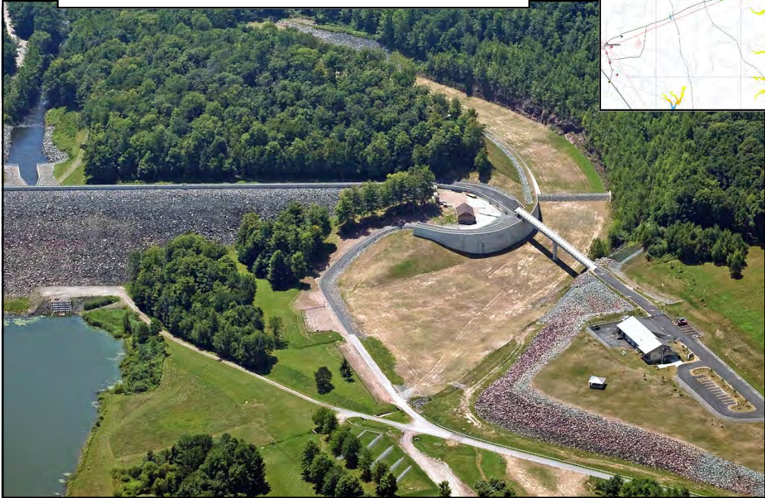
Prompton Lake, Lackawaxen River Basin, PA: Recent major modifications included an enlarged spillway, a protective concrete wall along the dam crest, and a new visitor's center.
