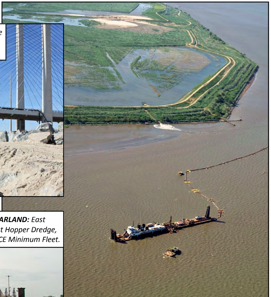
Delaware River Main Channel Deepening: Dredging south of Wilmington, DE for pumpout across the river to Killcohook Island Confined Disposal Facility under the first deepening contract in 2010.
