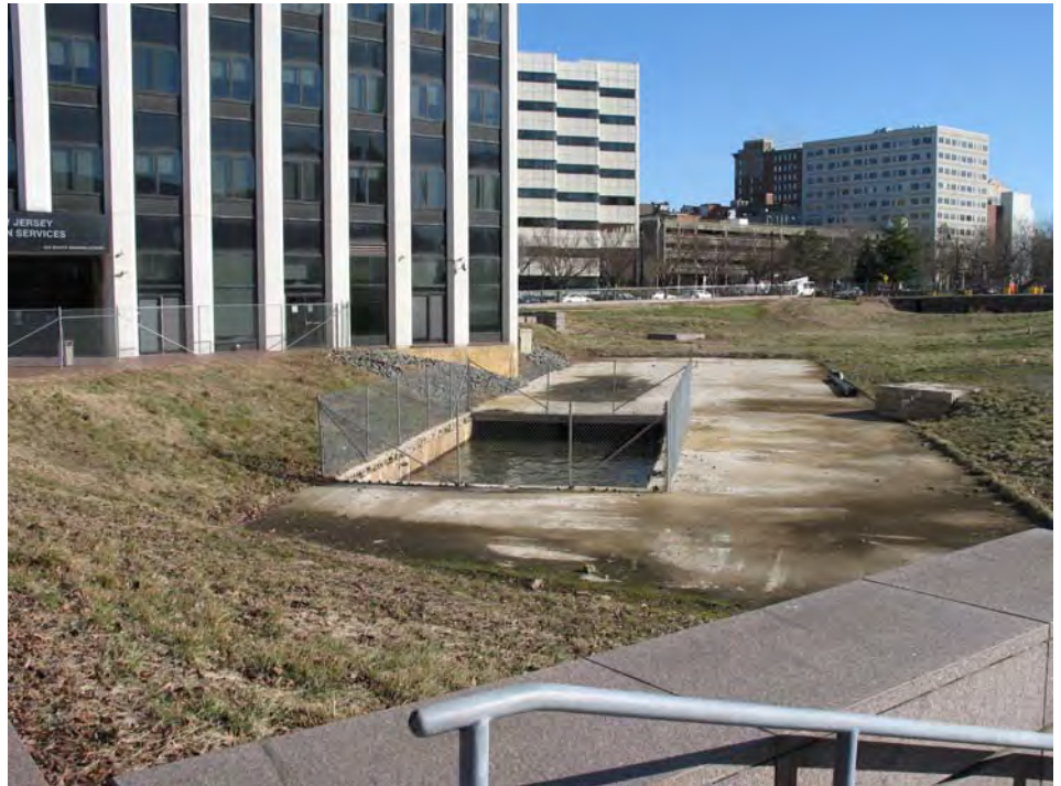
View of existing creek culvert looking upstream toward the historic Broad Street Bridge in downtown Trenton, NJ
