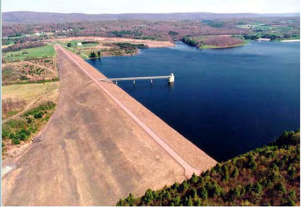
The project consists of an earth and rock filled dam; a spillway around the north end of the dam; and gate controlled outlet works discharging through a conduit on rock along the right abutment.
