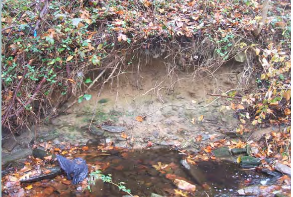
Eroding stream banks are a prevalent issue within the Wissahickon Creek watershed, making stabilization an important measure under consideration.
