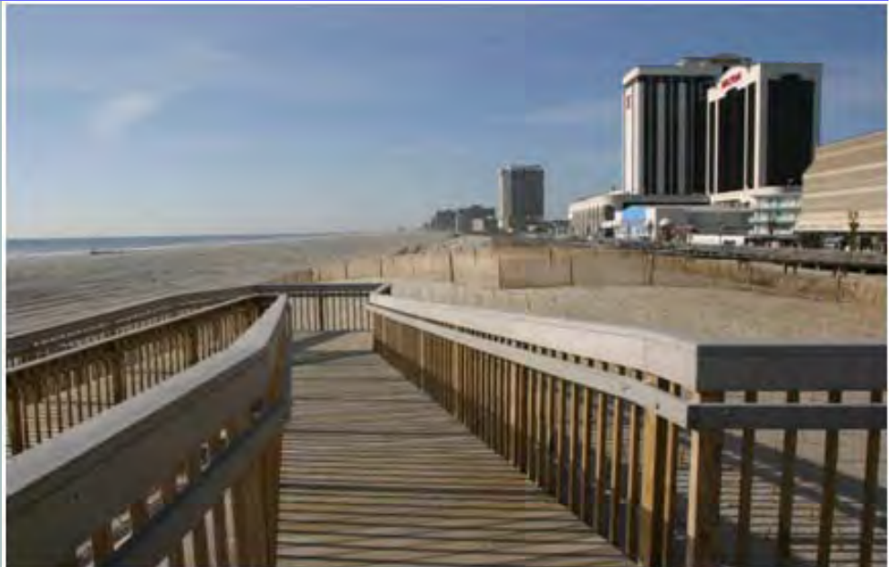
Absecon Island - Completed Handicap Dune Crossing.
