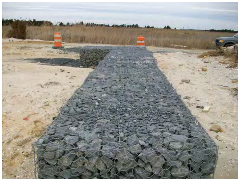
Completed section of gabion wall.
