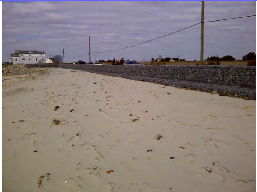
Completed gabion revetment with restored beach.
