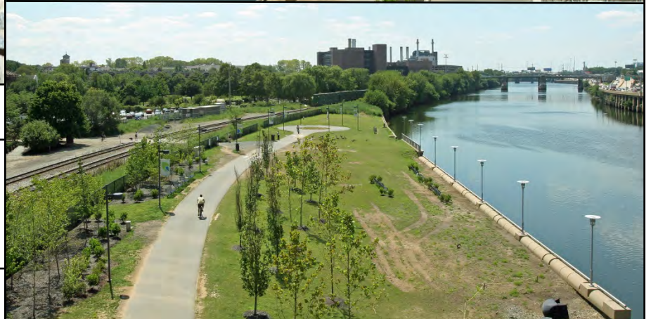
Schuylkill River Park, Philadelphia, PA: Construction of this multi-use linear park added highly visible and accessible green space in the heart of the city.
