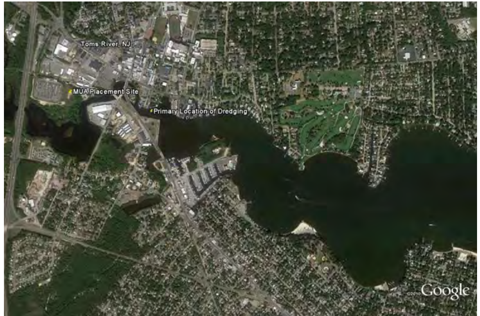
Aerial view of project area—Toms River, NJ
