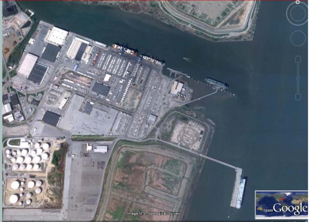
The project extends from the confluence of the Delaware River and the Christina River upstream, a length of about 9.9 miles. It is located 65 miles from the Atlantic Ocean. The photo shows Wilmington Harbor.
