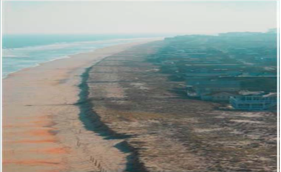
The plan includes dune grass, dune fencing, and suitable advance beach fill and periodic nourishment every four years to ensure the integrity of the design. Photo of Fenwick Island looking South.
