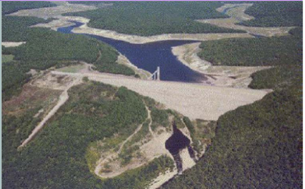
Francis E. Walter Dam and Reservoir
