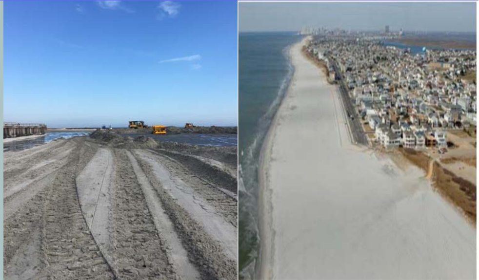
Left: Beachfill construction near 15th Street North in February 2018.
