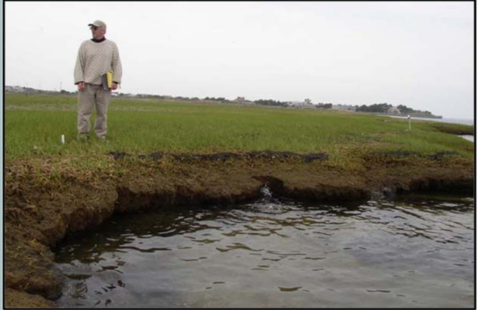
Mordecai Island is located west of Long Beach Island near Beach Haven Borough, New Jersey and is adjacent to the New Jersey Intracoastal Waterway (NJICW), the main navigation channel of Barnegat Bay. Erosion along the coastline pictured above.
