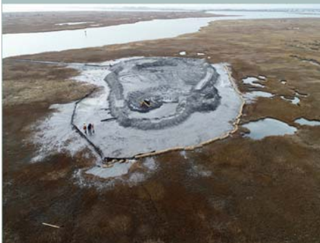
Habitat Creation at Great Flats, near Stone Harbor NJ conducted as part of the NJIWW dredging and beneficial use placement project in December 2018.. Barnegat Bay Dredging from Harvey Cedars, NJ was contractor for this and several innovative placement projects done through collaboration with the State of NJ.
