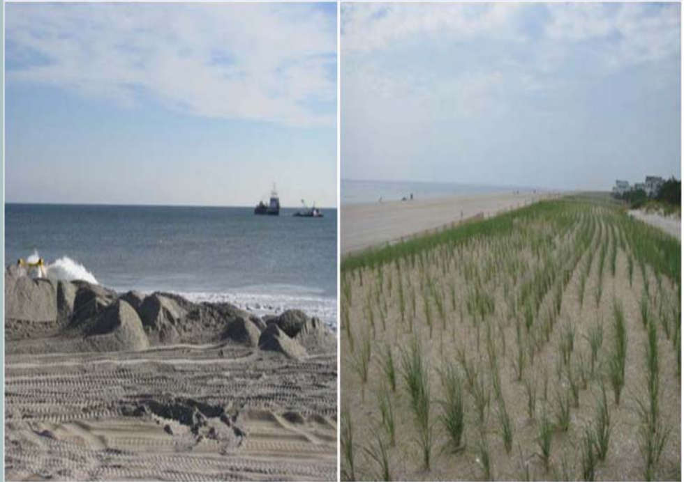
Left: Harvey Cedars Beach fill Initial Construction Right: Harvey Cedars Completed Dune Section
