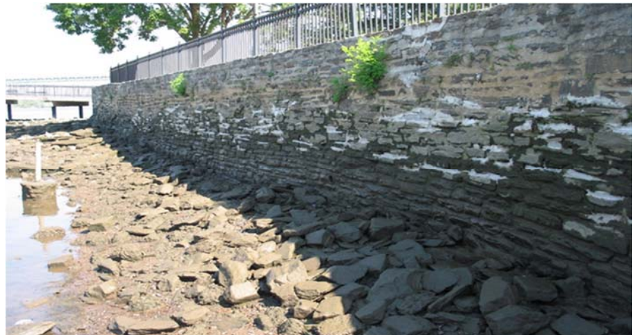
View of seawall with recent local repairs
