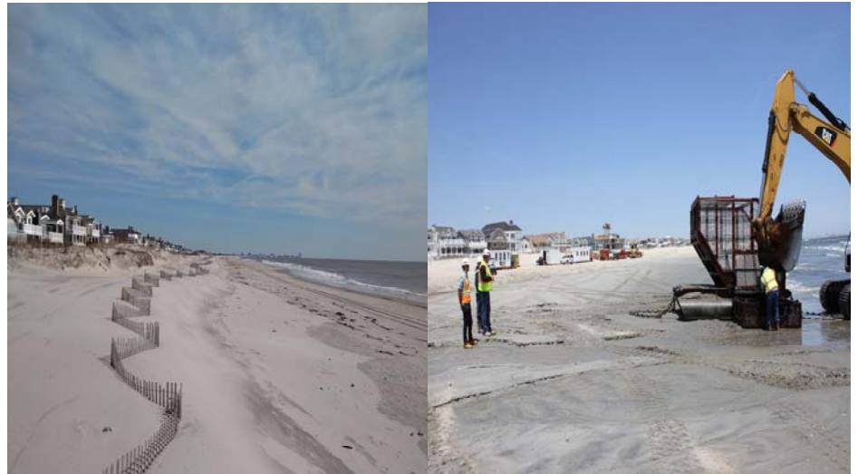
Preconstruction & during construction
