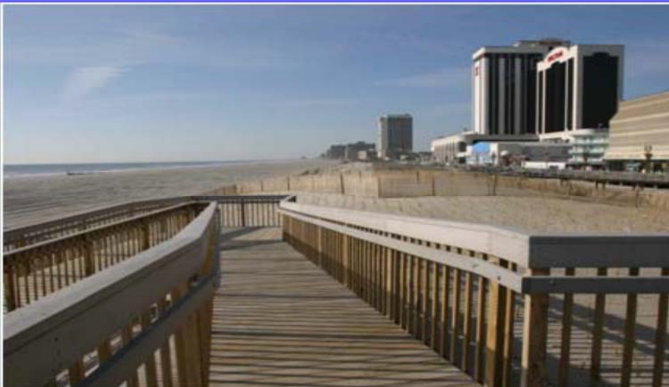
Absecon Island - Completed Handicap Dune Crossing.
