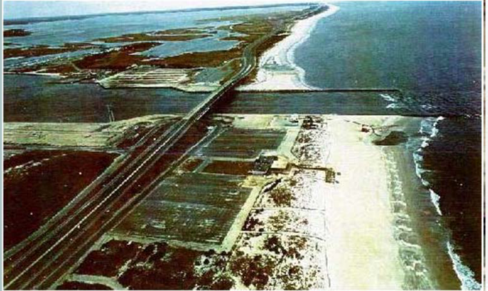
Indian River Inlet, Delaware, looking to the north showing the portable sand bypass system excavating a hole in the south fillet at the inlet. The system consists of a crane that holds an educator pump that removes sand from the beach face, two pumps to move the sand over the bridge, and a discharge line on the north side that discharges the sand onto the beach (where it looks wet in the photo).
