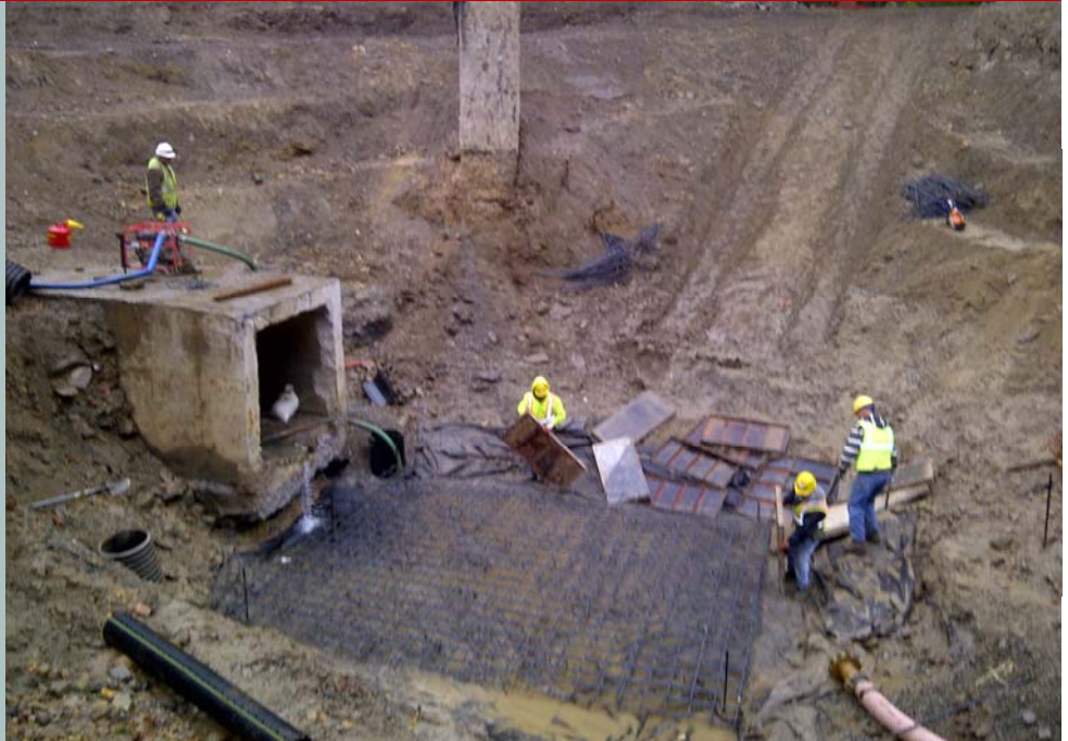
Construction of a vault structure to control sewer overflow along Indian Creek in Philadelphia as part of the Cobbs Creek Habitat Restoration project in 2013.
