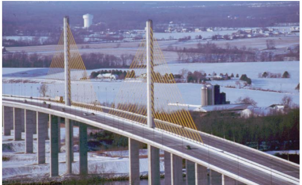
Senator Roth Bridge (SR-1).
