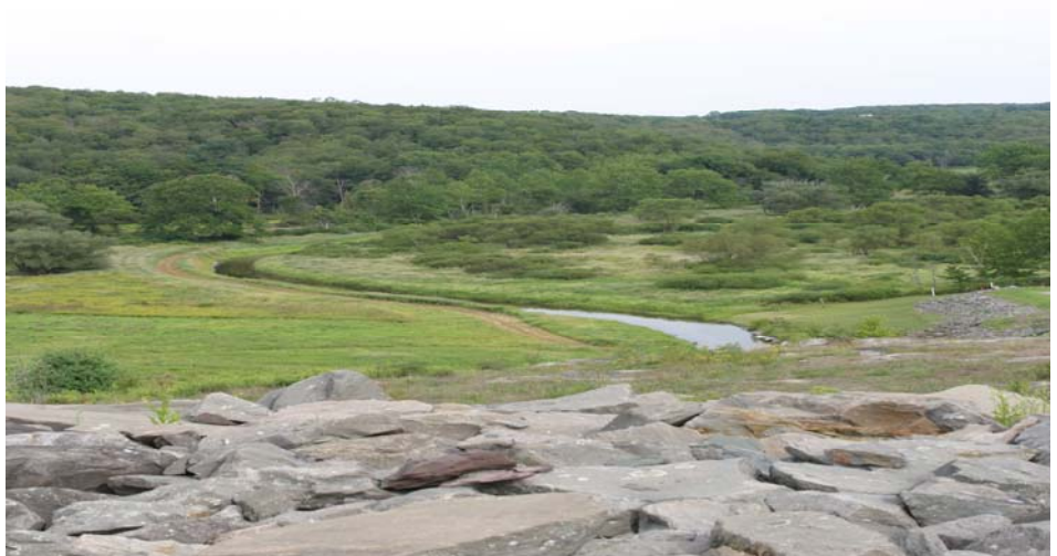
Dyberry Creek at base of General Jadwin Dam.
