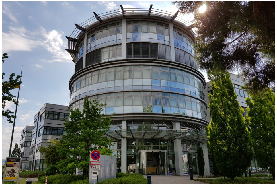
SAP Headquarter Campus in Walldorf Germany is home to the Dell Technologies Global SAP Center of Excellence
