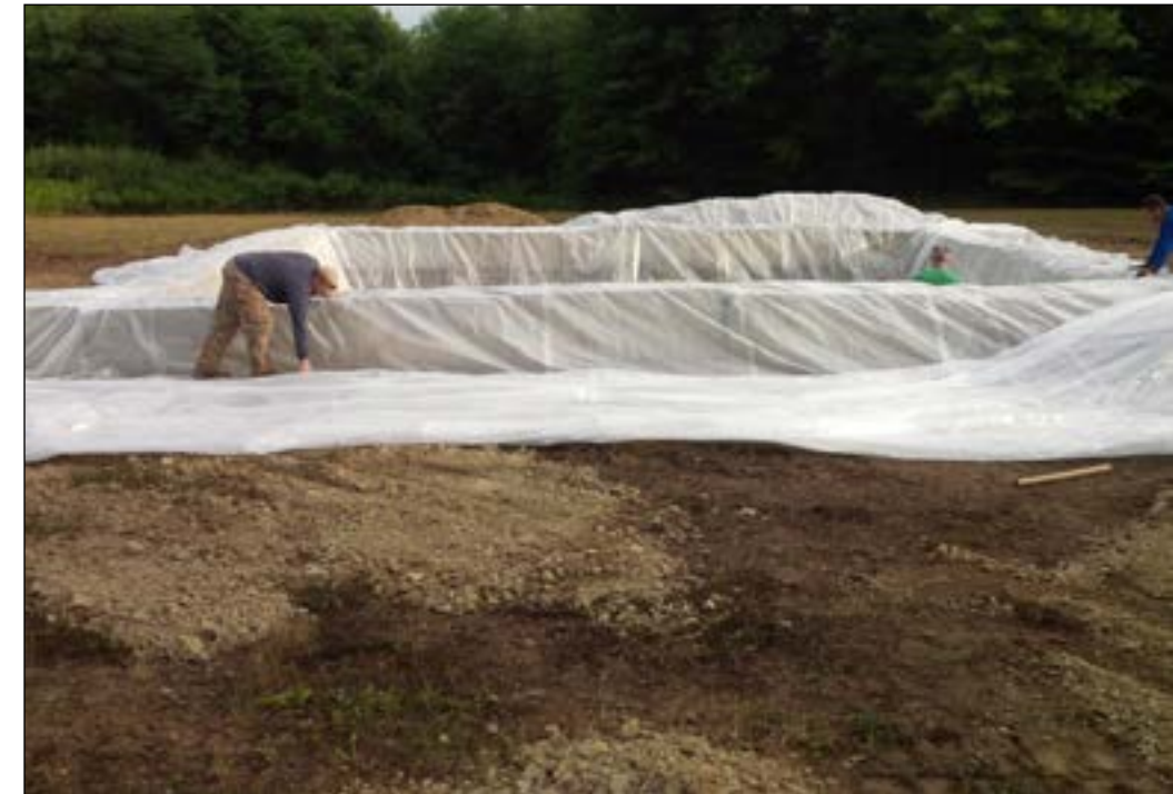
Permanent BEM liner being prepared for use at Camp Ravenna, Ohio.
