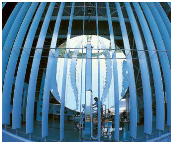
Figure 3: The solar furnace at the Solar Technology Laboratory of the Paul Scherrer Institute: a sun-tracking heliostat on-axis with a paraboloidal reflector delivers concentrated solar energy at peak radiative fluxes exceeding 5,000 suns (1 sun = 1 kW/m 2 ).
