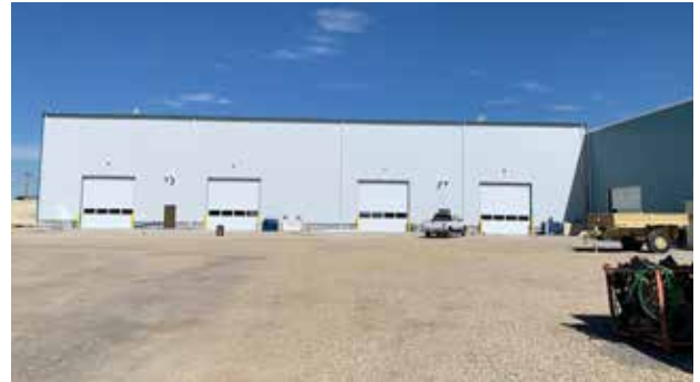
Top down: Inside the new 12,390 sq. ft. maintenance bay, showcasing the 10-Ton crane, which spans the entire length of the shop. Updates to this facility provide adequate space to service all current vehicles with room for future maintenance needs. Outside the Unit Training Equipment Site at Camp Williams. This project consolidated existing bays and added a new 12,390 sq. ft. maintenance bay among many other significant upgrades.
