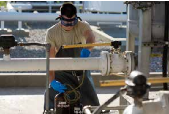
Above: Master Sgt. Robert Zepeda, left, and Airman 1st Class Andrea Reyes secures energy dispersing pads to a 463L aircraft pallet during a cargo build-up exercise July 30, 2019. Below: Airman 1st Class Hans Grow draws jet-fuel samples during tank truck receipt in the fuels yard for laboratory analysis in August 2019.
