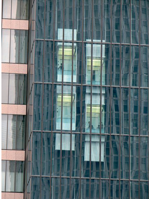
Fig 1: Double elevator at Midland Square Nagoya, Japan (taken from [WC16])
