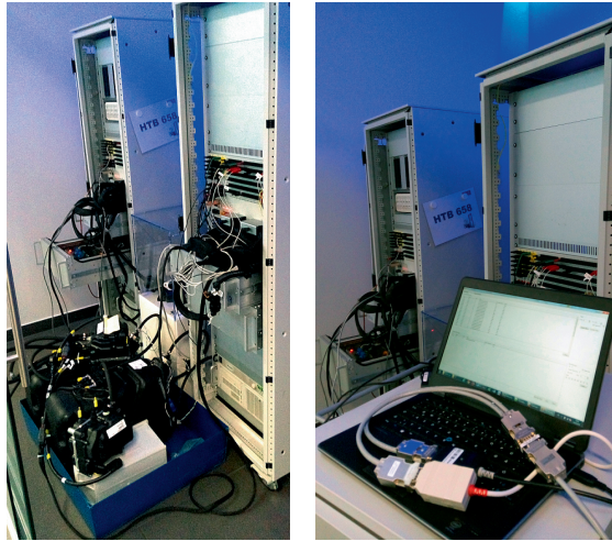
(a) Photo of a heavy duty vehicle Hardware-in-the-Loop System setup (b) Connecting CAN-CT via the PCAN-USB adapter
