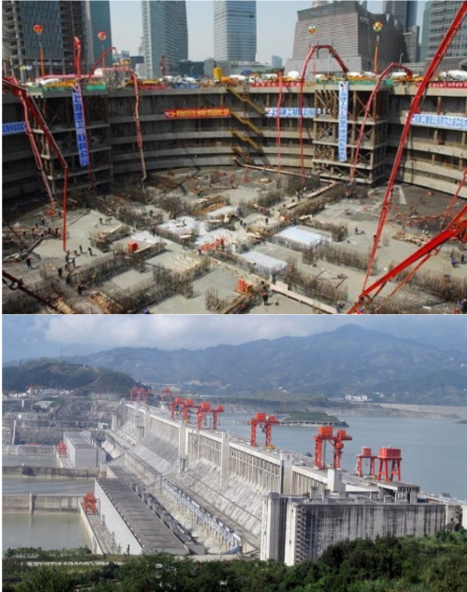
Figure 1.1: Slag blended cement used in the foundation of Shanghai Tower of China (top) [8], and fly ash blended cement used in Three Gorges Dam of China (bottom) [9].
