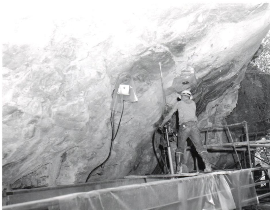
Figure 9. Cowin and Co. employees installing roof bolts. (Photo courtesy NPS, RUCA 1966).
