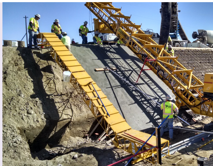
LEVEE CONSTRUCTION IN PUEBLO, COLORADO
