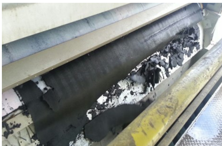
Image: Solid removal of dewatering system (Source–Green Mark Projects Sdn. Shd.).
