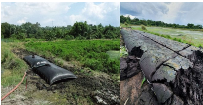
Image: (Left) C-tube filling process and (right) dry solid captured (Source–PT. Elmoz Geo Solusi).
