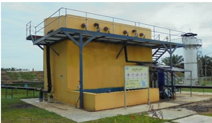
Image: BPO H 2 S biogas scrubber at PT. Harapan Sawit Lestari (Source–BPO).
