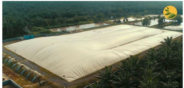
Image: Biogas plant at Sinarmas, Central Kalimantan (Source—Organics Bali).
