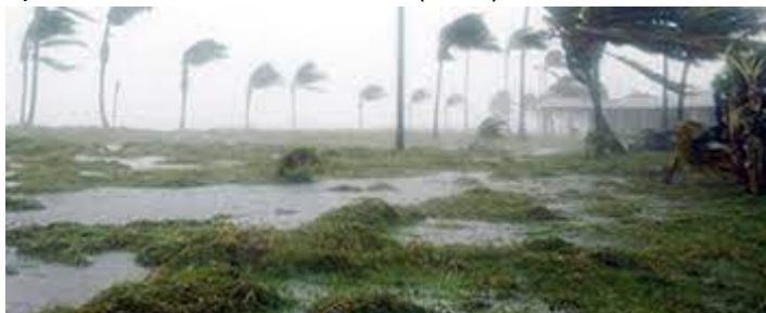
Hurricane Laura was a category 4 storm that caused 20 deaths and damaged buildings, roads and infrastructure with its 150 mph sustained winds and widespread flooding in August 2020.
