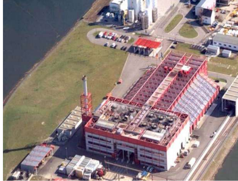
Thermoselect Gasification Incinerator
