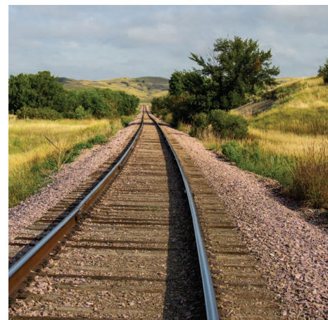
The MRC line west of Chamberlain before (top) and after (bottom) rehabilitation.
