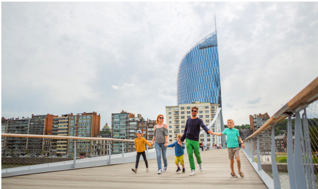
The new bridge for pedestrians and cyclists in Liège, city center. Photo: © WBT, Denis Erroyaux
