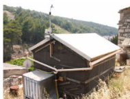
Dew collection roof retrofit
