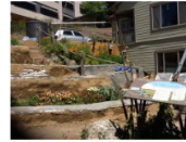
Plastering CCAT Earthbag Terrace
