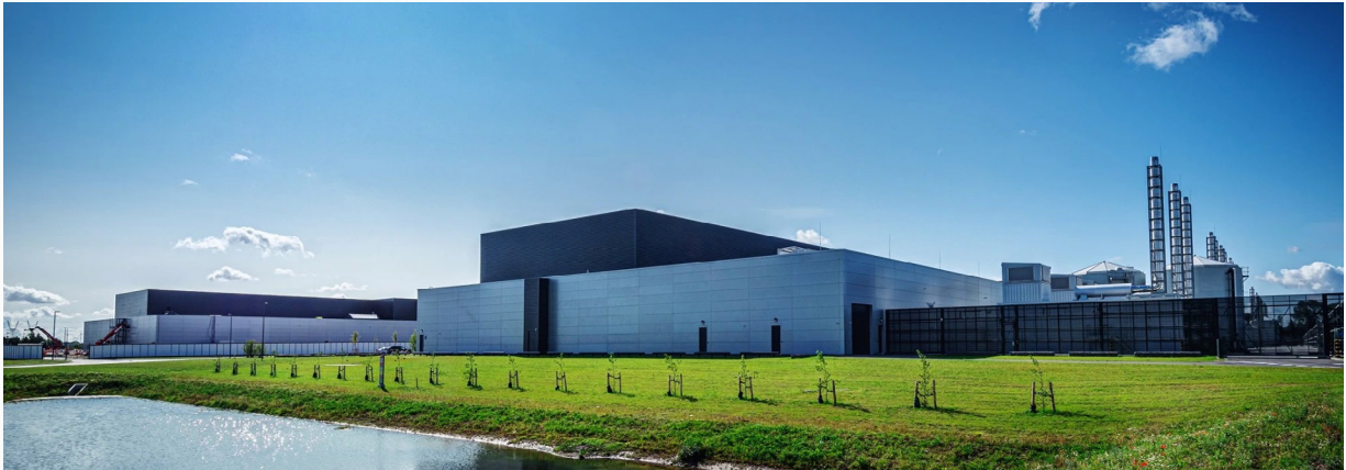
Our data center in Odense, Denmark includes a system that reuses excess heat from data halls to warm homes in a neighboring community. We were able to divert 90 percent of the construction waste footprint from landfills through reuse, recycling and waste-to-energy facilities, and the project won the 2020 Data Center Dynamics "Hyperscale Data Center Innovation Award"
