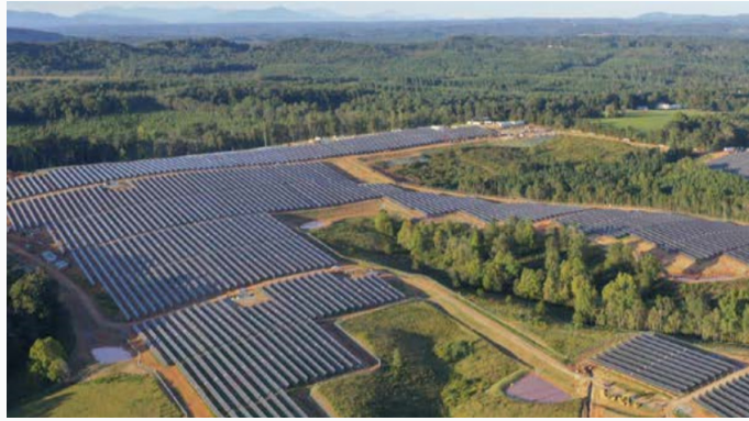
61.6 MW Altavista Solar Project in Virginia
