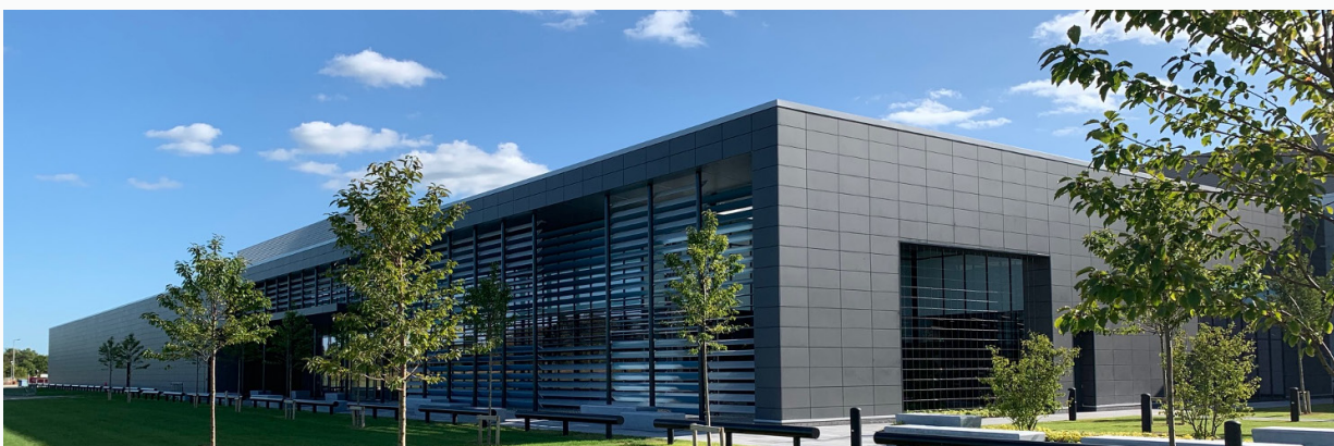
In 2020, we earned LEED Gold certification for our third data center building (CLN3) at our Clonee, Ireland campus.
