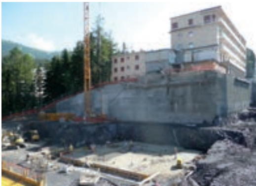
Complex excavation safety – reinforced and prestressed shotcrete wall
