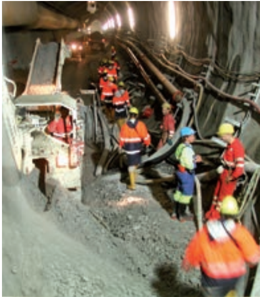
Excursion to the construction site of the Gotthard base tunnel
