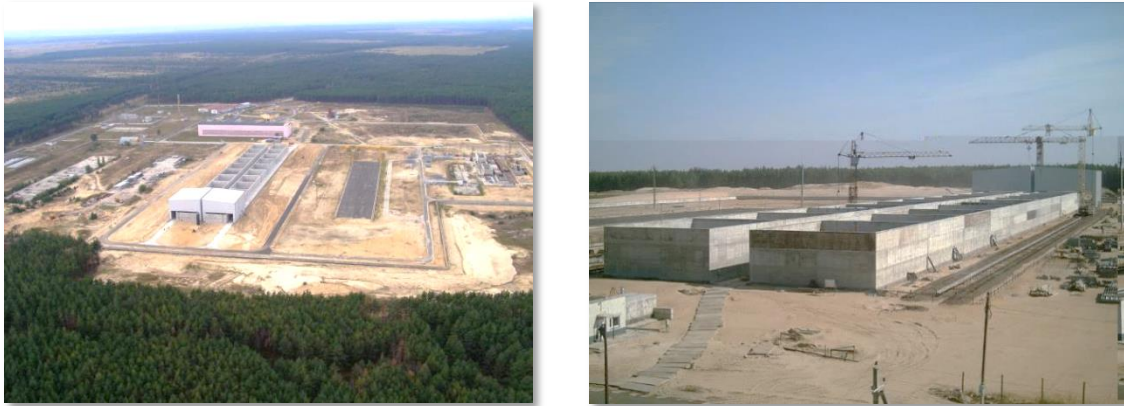
Figure 8.2. The Engineered Near-surface Disposal Facility
