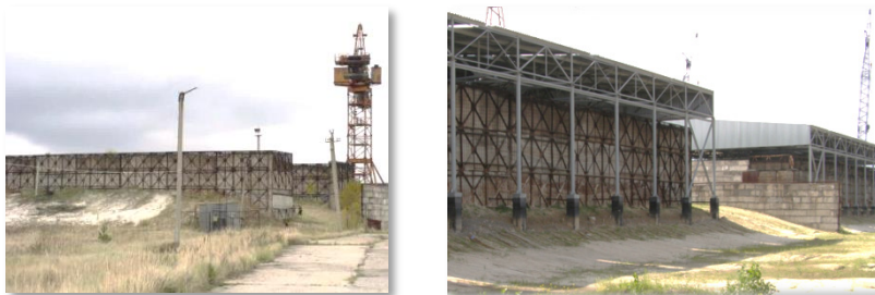
Figure 4.1. SDRW “Pidlisny”: Before and after reparation works
