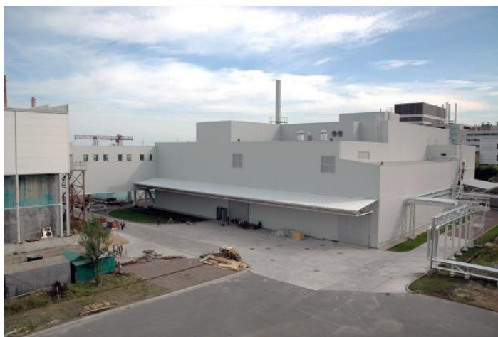
Figure 7.7. Solid waste processing facility
