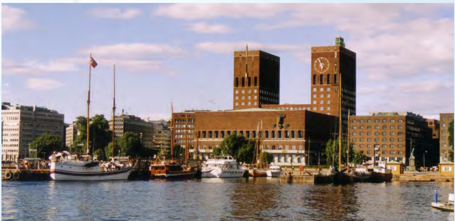
Oslo town hall and harbour
