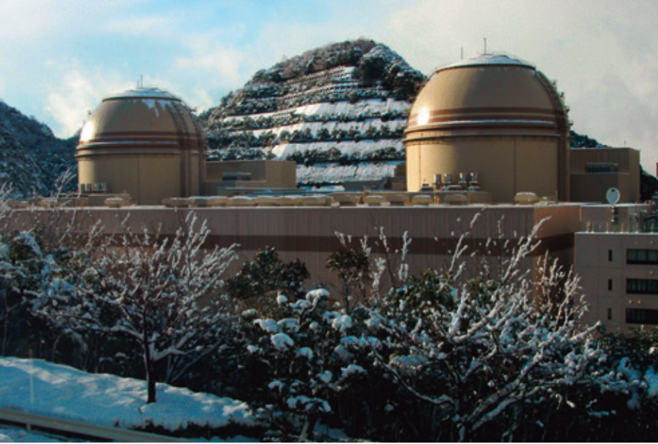
Ohi Nuclear Power Plant, units 3 and 4, Japan. Wikimedia Commons
