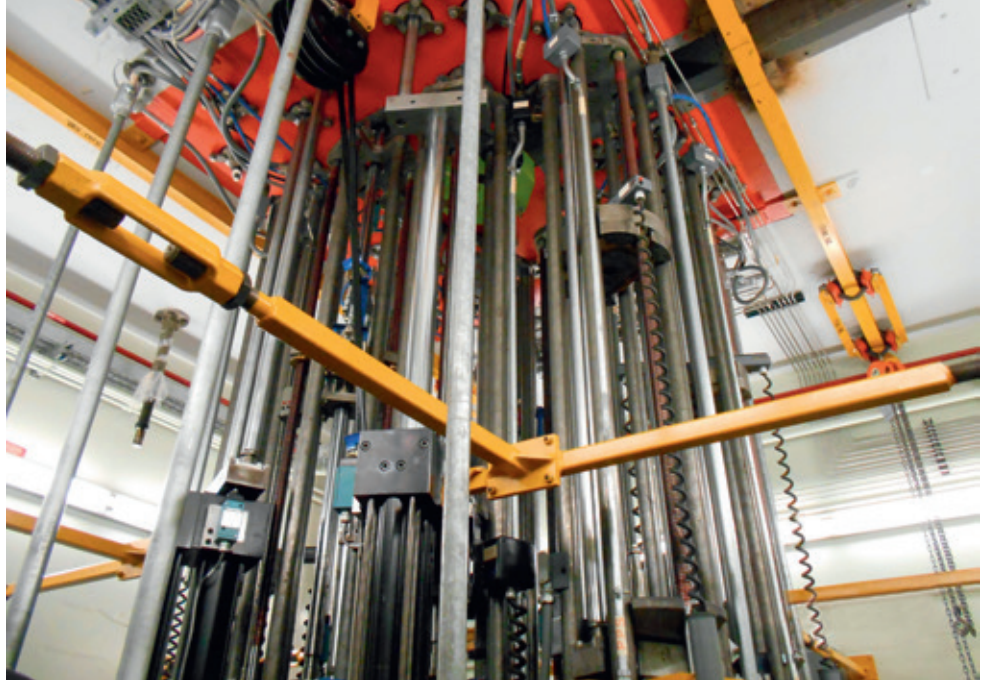
TREAT subpile room, United States. © Rsb8382
