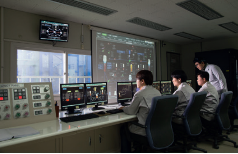
The ATLAS facility. KAERI, Korea
