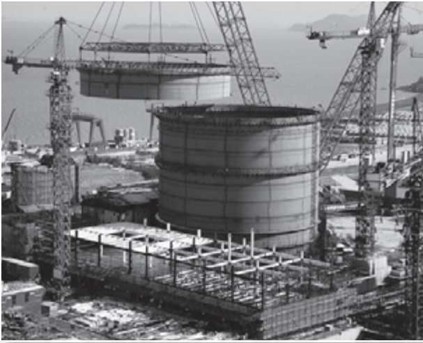
An AP1000 under construction.
