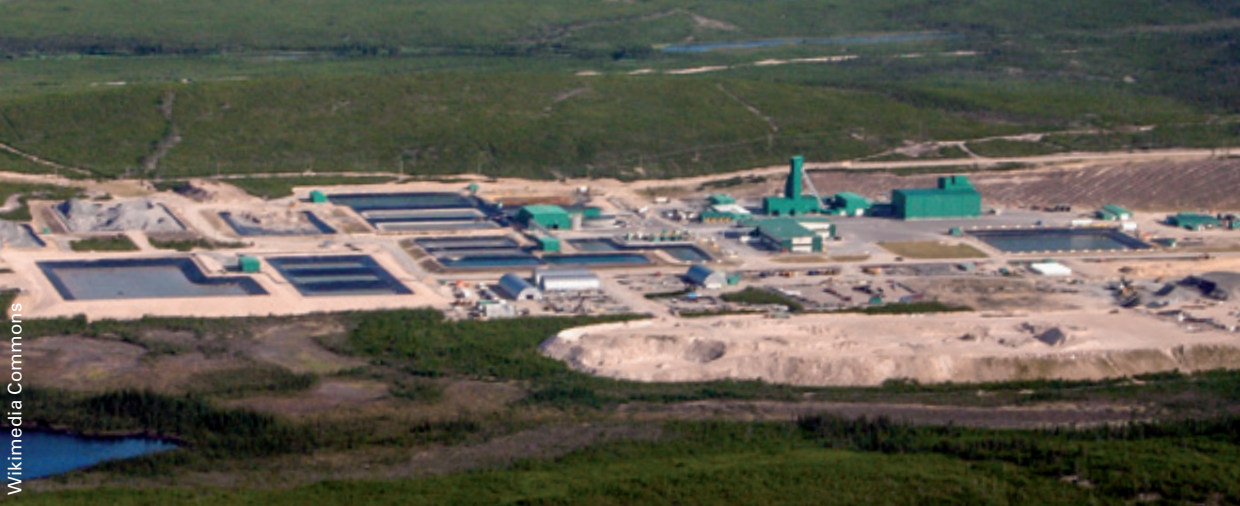
Aerial view of the McArthur River uranium mine, Canada.
