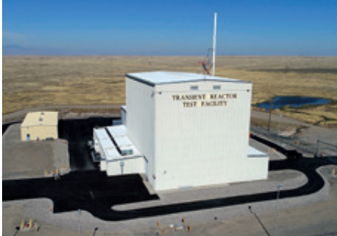
The Transient Reactor Test (TREAT) Facility located at the INL Materials and Fuels Complex.
