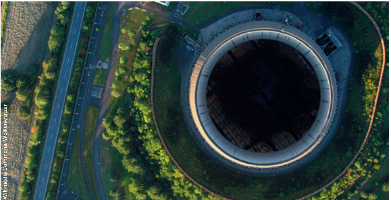
Vertical view of a cooling tower at a nuclear power plant.
