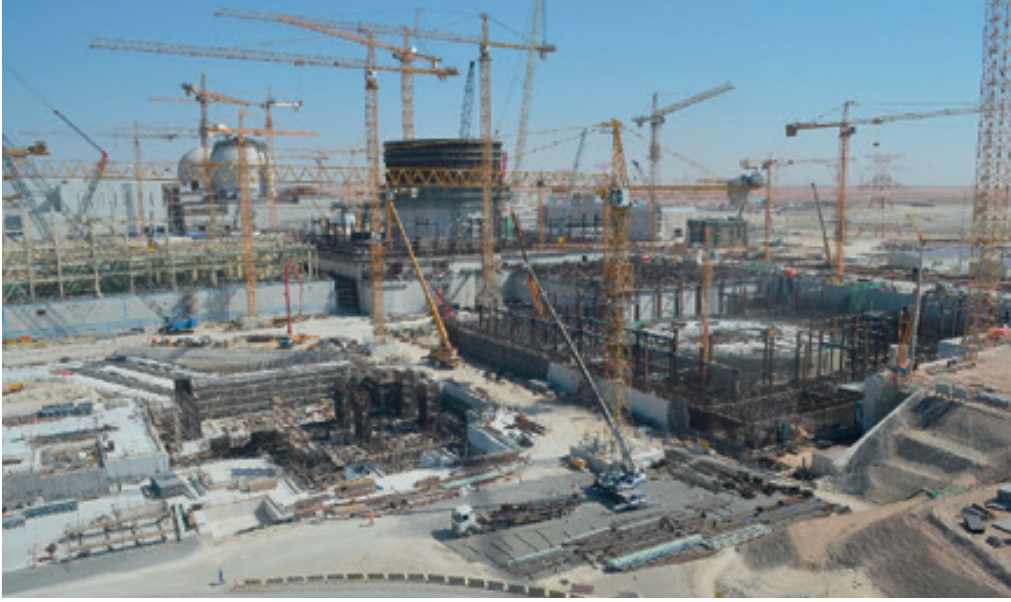
Barakah NPP, units 3 and 4, United Arab Emirates, September 2016.
