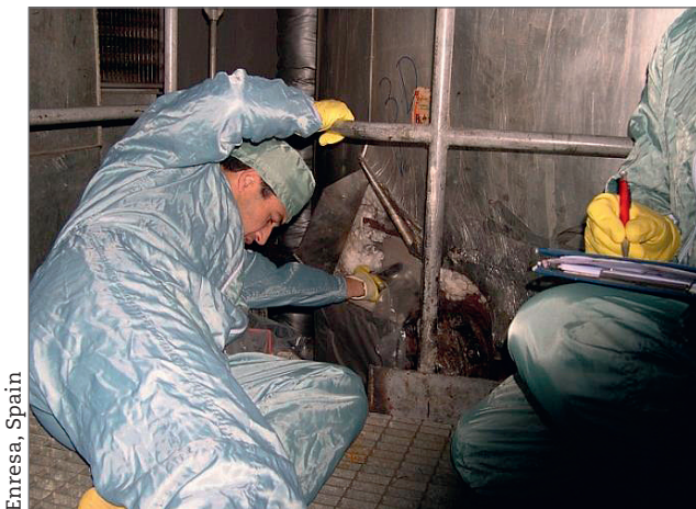
Steam generator radiological characterisation (left) and dismantling of elements from the primary pump (right), José Cabrera nuclear power plant, Spain.
