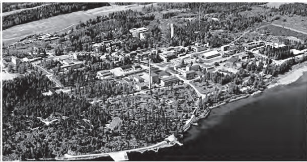
The Studsvik site where the workshop was held.
