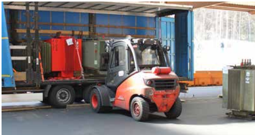
Figure 12: Transport of transformers to recycling facility
