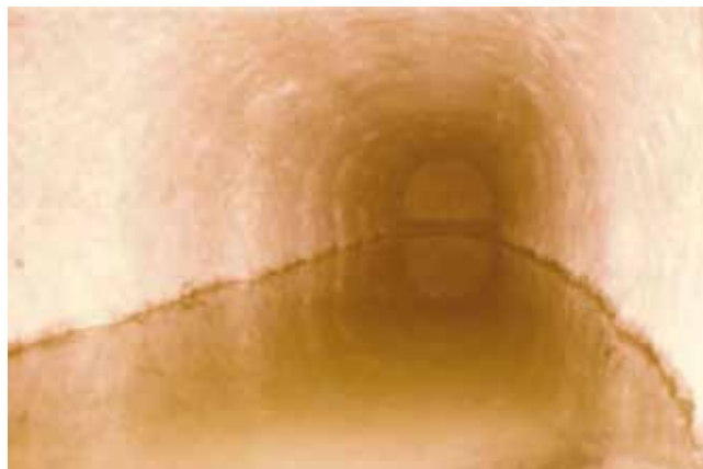
Figure 5: Brine from cavern leaking in Asse mine
