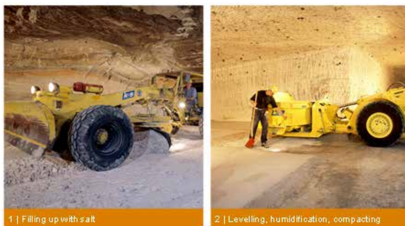
Figure 7: Mining – roadway construction
