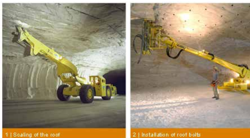
Figure 6: Mining – cavity preparation
