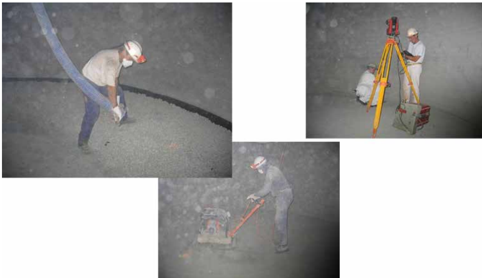
Figure 24: Building of bentonite seal
