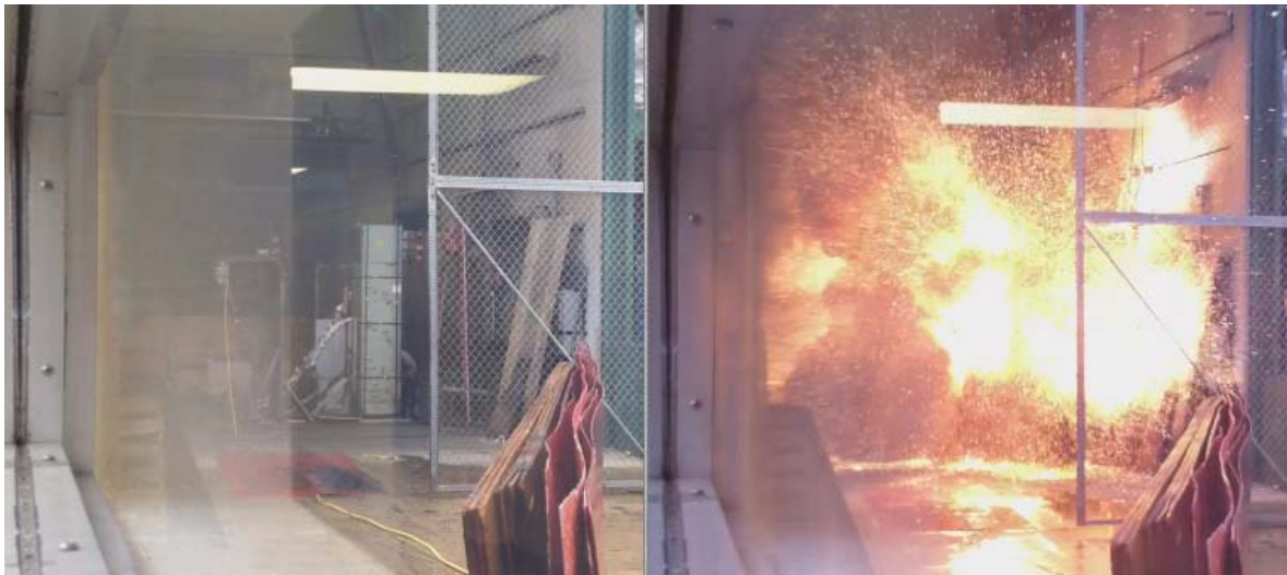
Figure 4. 480 V load center undergoing HEAF Testing: before arcing (left) after arcing (right)
